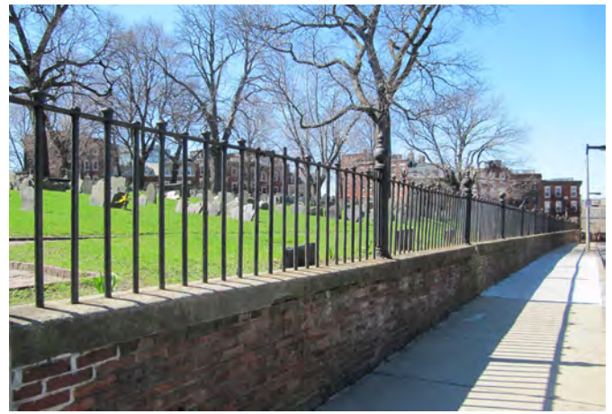
The Charter Street fence in 2012. Almost all of the finials are missing on this fence now.
