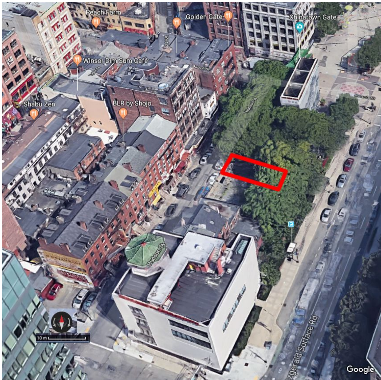
Figure 6- Google 3D aerial image showing project area (red) near gate and Soo Hoo park (upper right). Note buildings on opposite side of Hudson street (center/left), which would have been identical to 6 Hudson Street prior to demolition.
