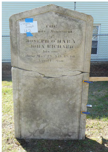
B.2: The bottom piece was set into the ground and the two pieces were attached together.
