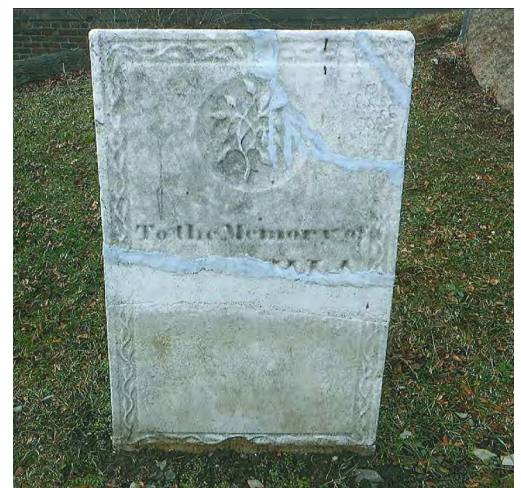
C.3: Since this headstone was missing its original bottom end, a new concrete base was attached with pins. The large top part was also pinned to the piece beneath it. Although the epitaph is missing, at least the remaining parts of the headstone are not lying on the ground.
