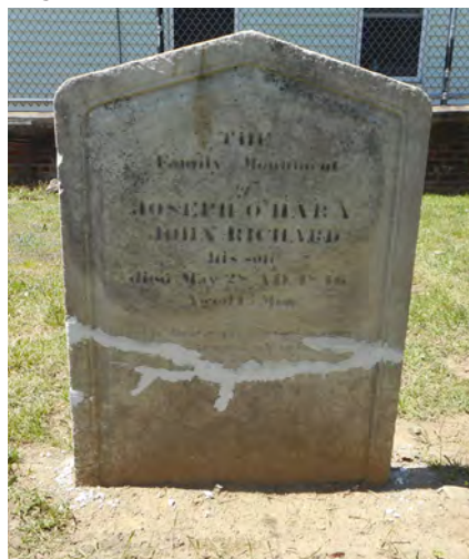
B.3: The gaps along the crack were grouted with a special repair mortar.
