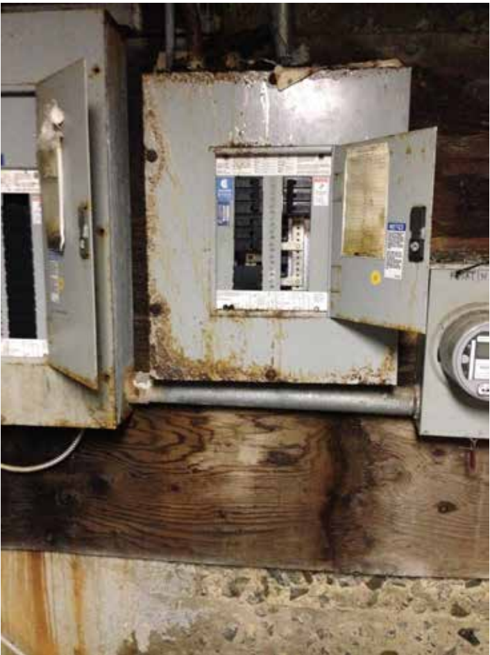
SERVICE PANELBOARD IN BASEMENT
