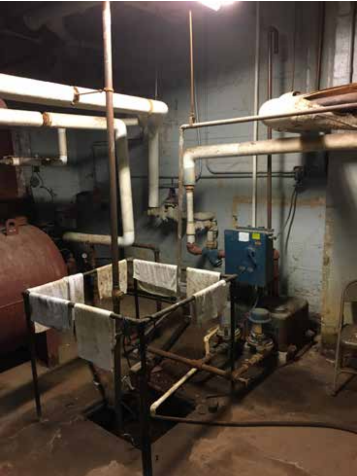
DUPLEX CONDENSATE PUMP UNIT
