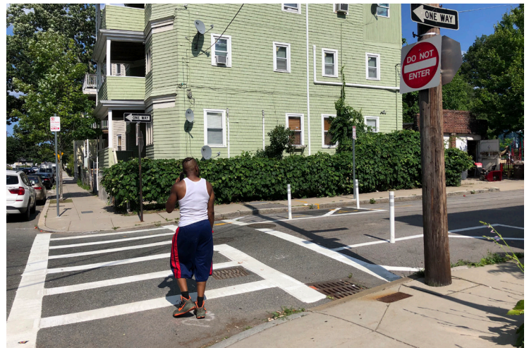
Photo: “Daylighting” with flexposts + paint
