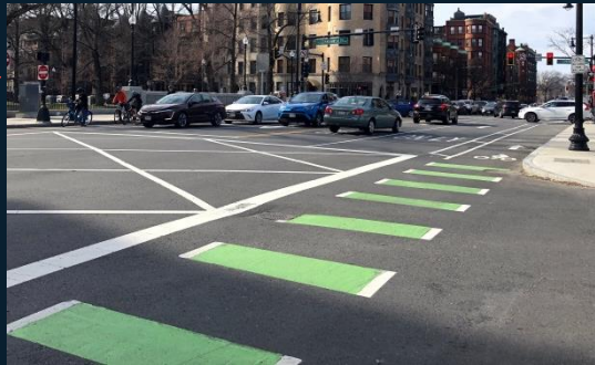
Intersection markings to highlight bike lane
