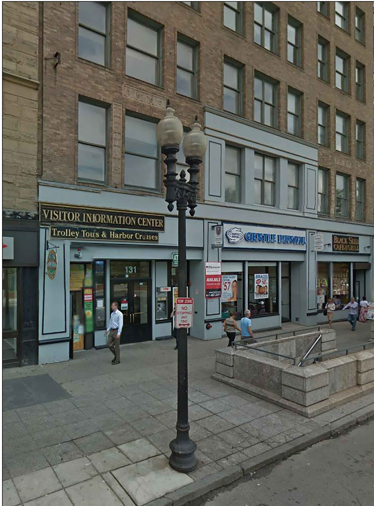
EXISTING PHOTOGRAPHIC VIEW
