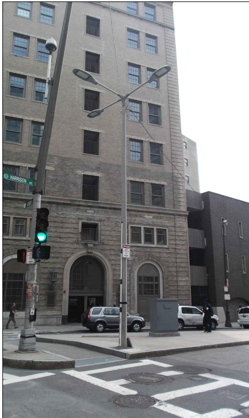
EXISTING PHOTOGRAPHIC VIEW
