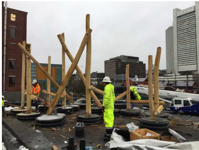
Log climber install
