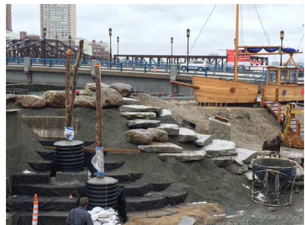
Locust posts/ stone scramble
