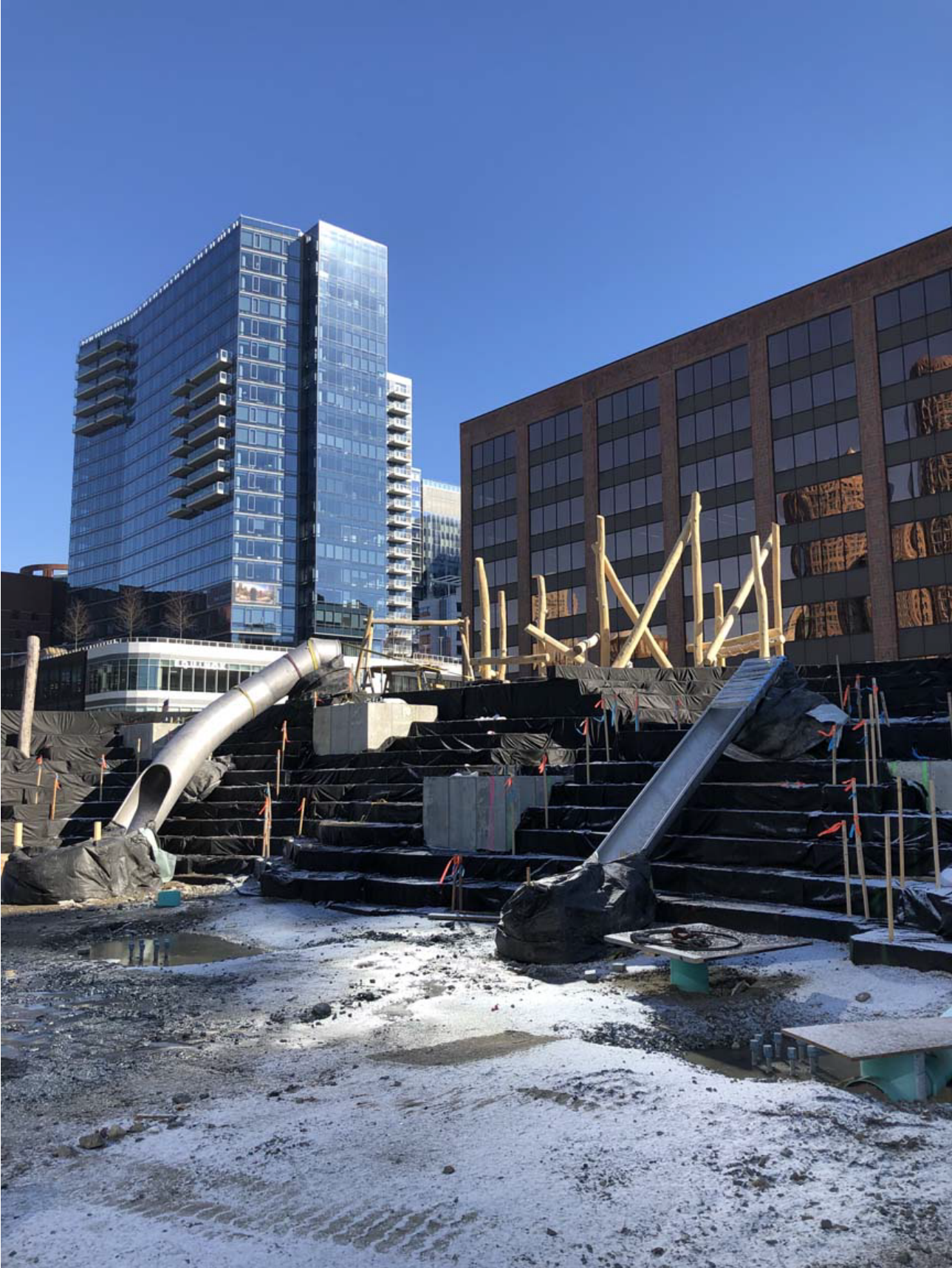
100% completion of geofoam/ slide install/ log climber install
