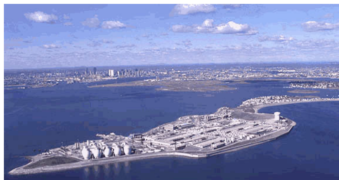
Deer Island Waste Water Treatment Plant
