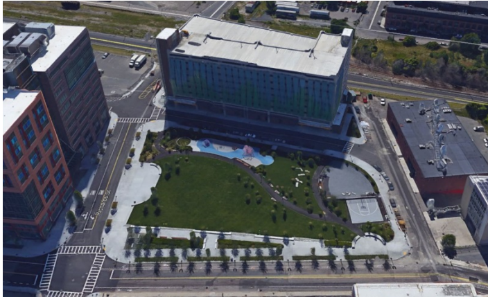
A Street Park at Richards Street, South Boston (Image Source: Google Earth)
