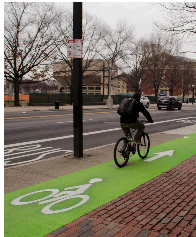
Vision Zero safety improvements on Massachusetts Avenue created better protected bike lanes. Photo credit: Toole Design Group
