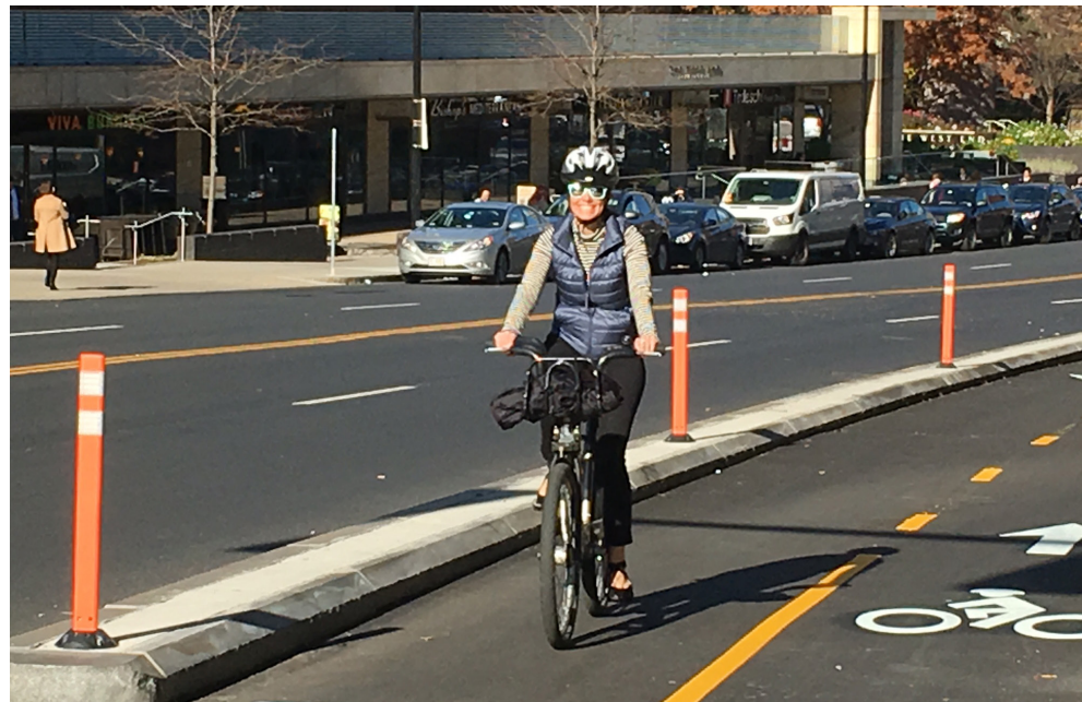
Protected bicycle lane on Staniford Street, Boston
