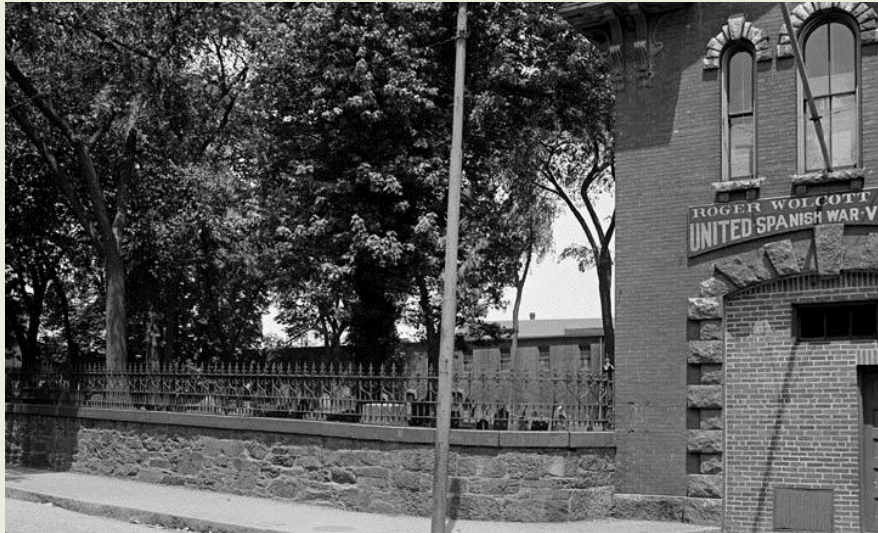
The highly ornamental fence shown in this photo from the 1920s was replaced by a plain fence.
