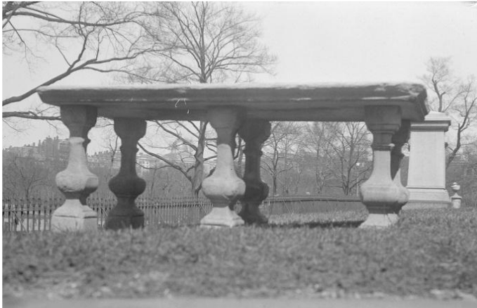
This old photo from Central Burying Ground shows what some table tombs used to look like. Frequently the carved legs deteriorated and were replaced by a rectangular brick base. Photo courtesy of the Boston Public Library, Leslie Jones Collection.
