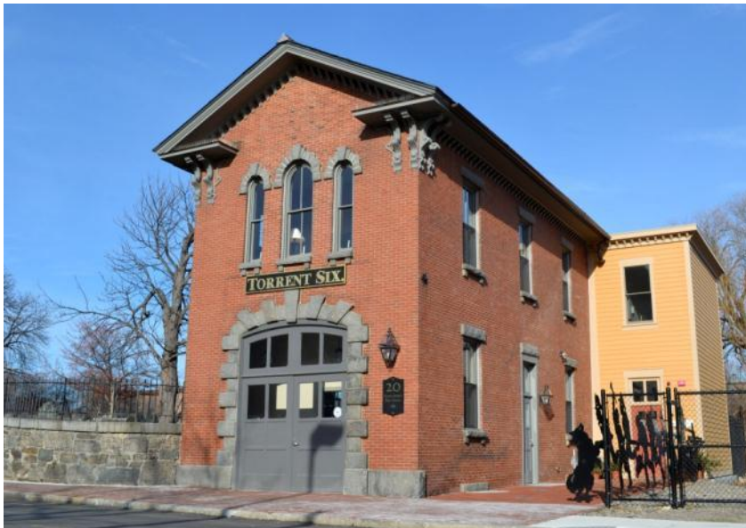
The beautiful building after renovation in January 2012.
