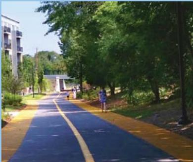
Bituminous Concrete Path with a Poured in Place Rubber Shoulder (Yellow Rubber)
