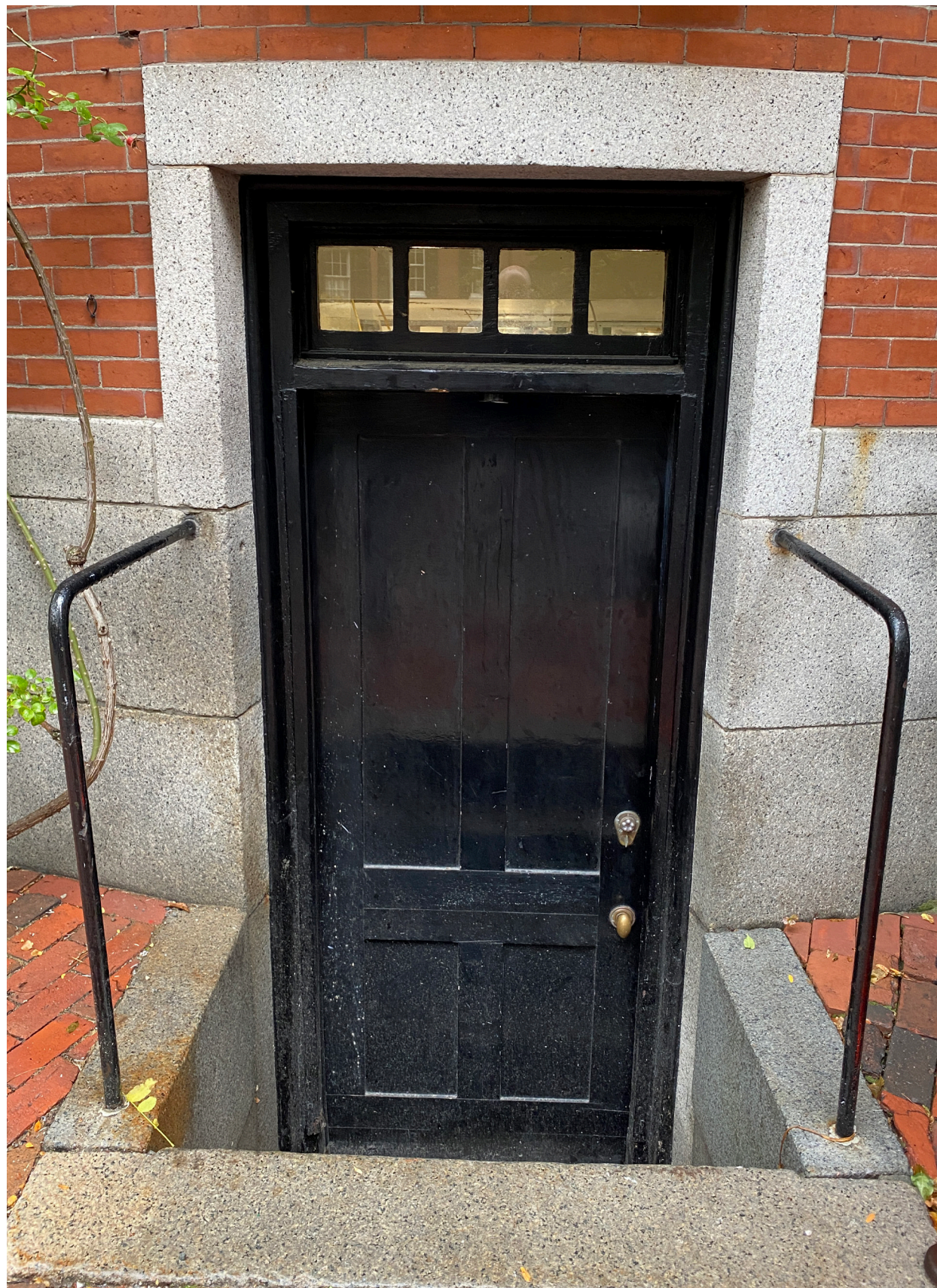
Existing Mudroom Door
