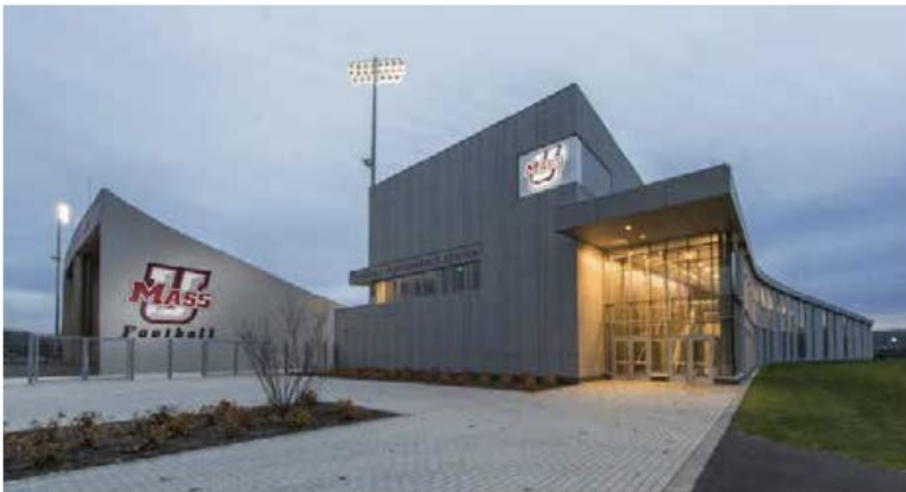
UMass Football Performance Center
