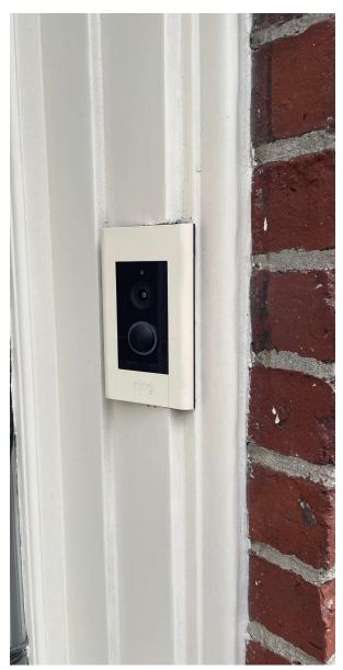
The current door bell was installed into the trim. The orientation of the device is angled to accommodate the wiring in the rear and allow for viewing who is at the door. The device is against the masonry behind the wood. We propose leaving the existing cover since it blends with the surround. The black crease slightly viewable along the perimeter would be painted to create seamless transition with the wood.
