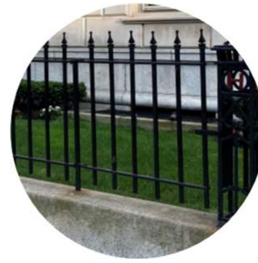
EXISTING WROUGHT IRON FENCE
