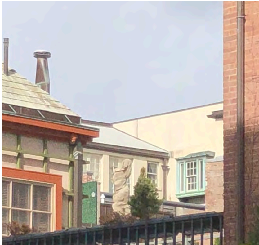
Magnified View #2 Showing Existing Courtyard Facade
