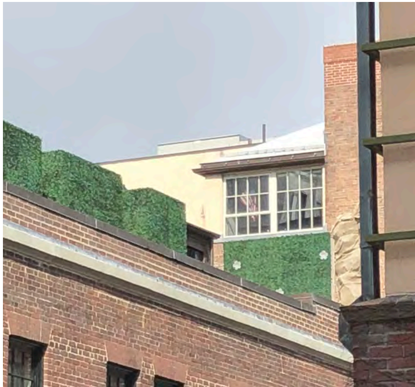
Magnified View #1 Showing Existing Courtyard Facade
