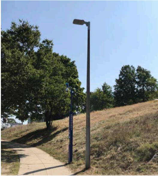
LIGHTING FIXTURE AND EMERGENCY TELEPHONE
