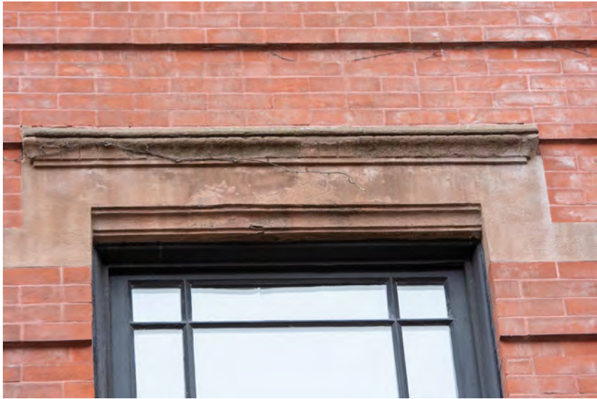
Brown stone and brick damage and staining detail
