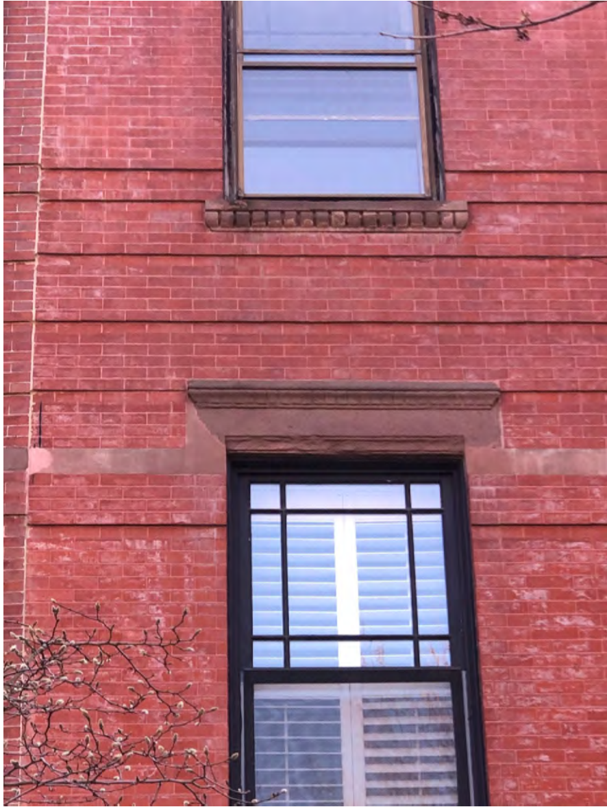
Brick efflorescence and staining
