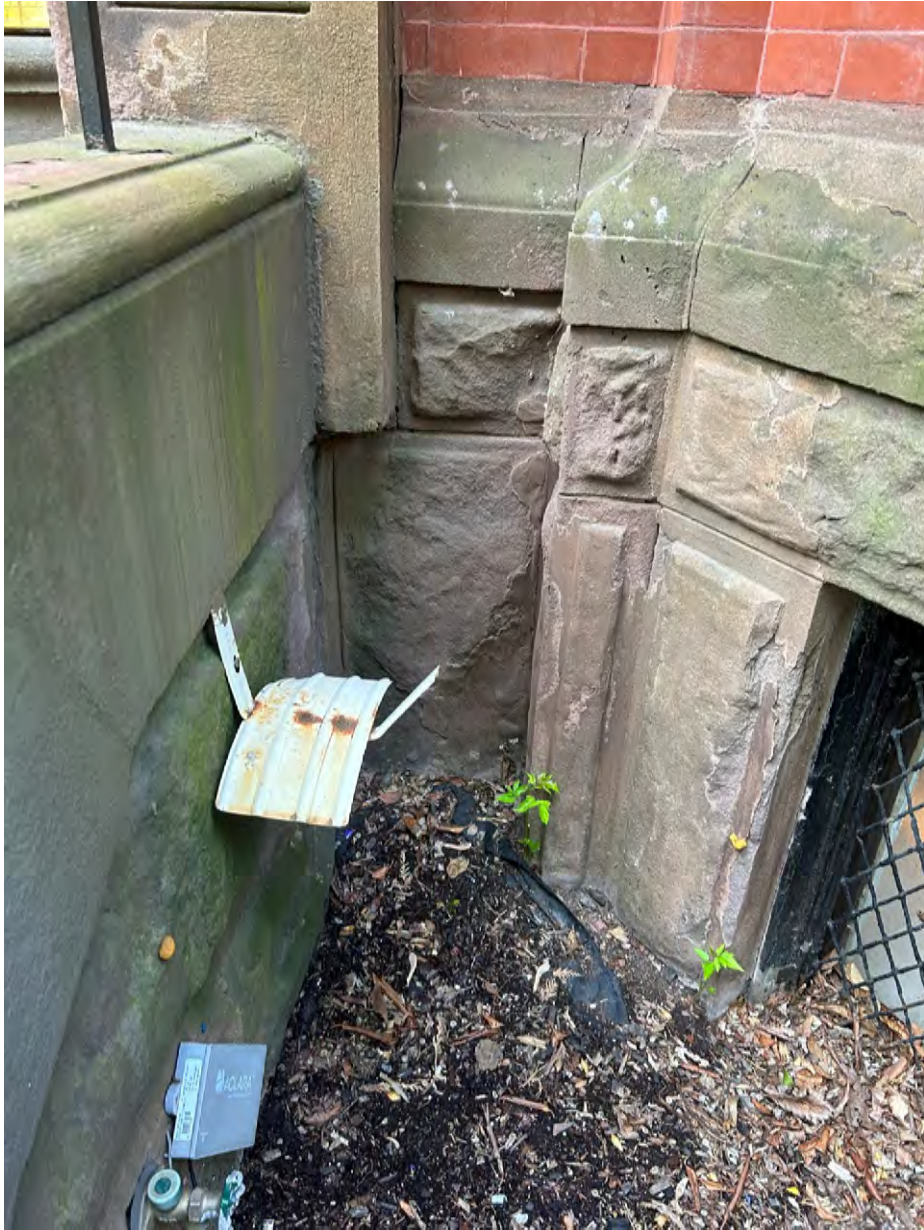
Front stair detail
