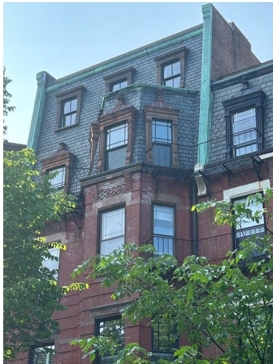
3 rd , 4 th and 5 th floor windows
