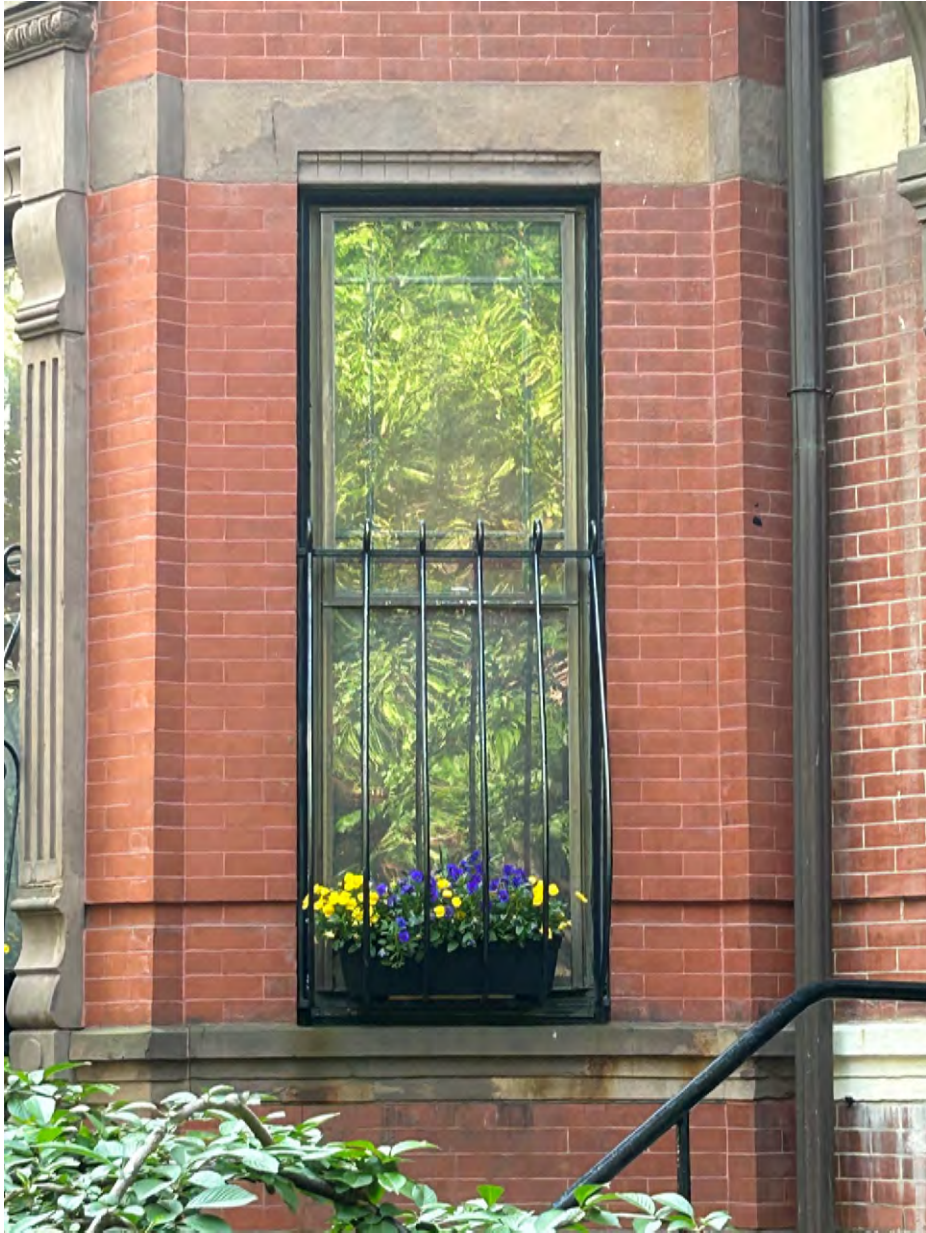
Bay window detail
