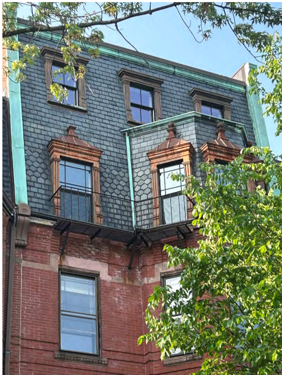
3 rd , 4 th and 5 th floor windows
