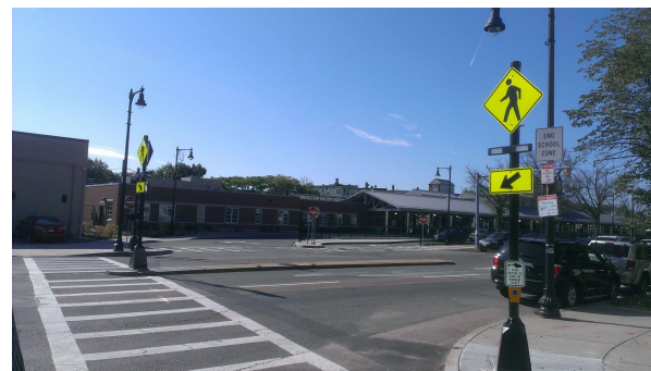
Pedestrian Rapid Flash Beacon
