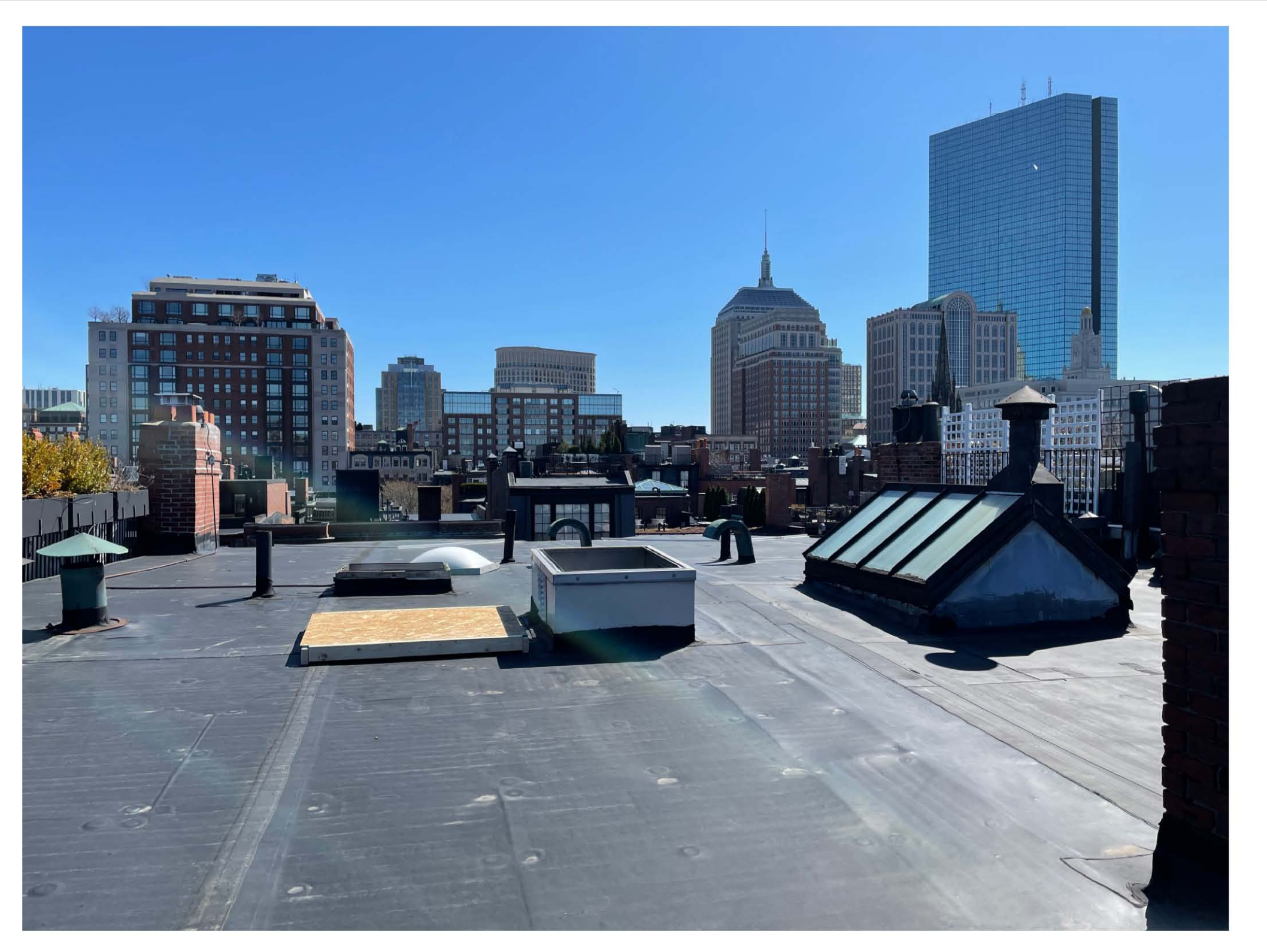
⑤ PHOTO OF EXISTING ROOF LOOKING SOUTH
