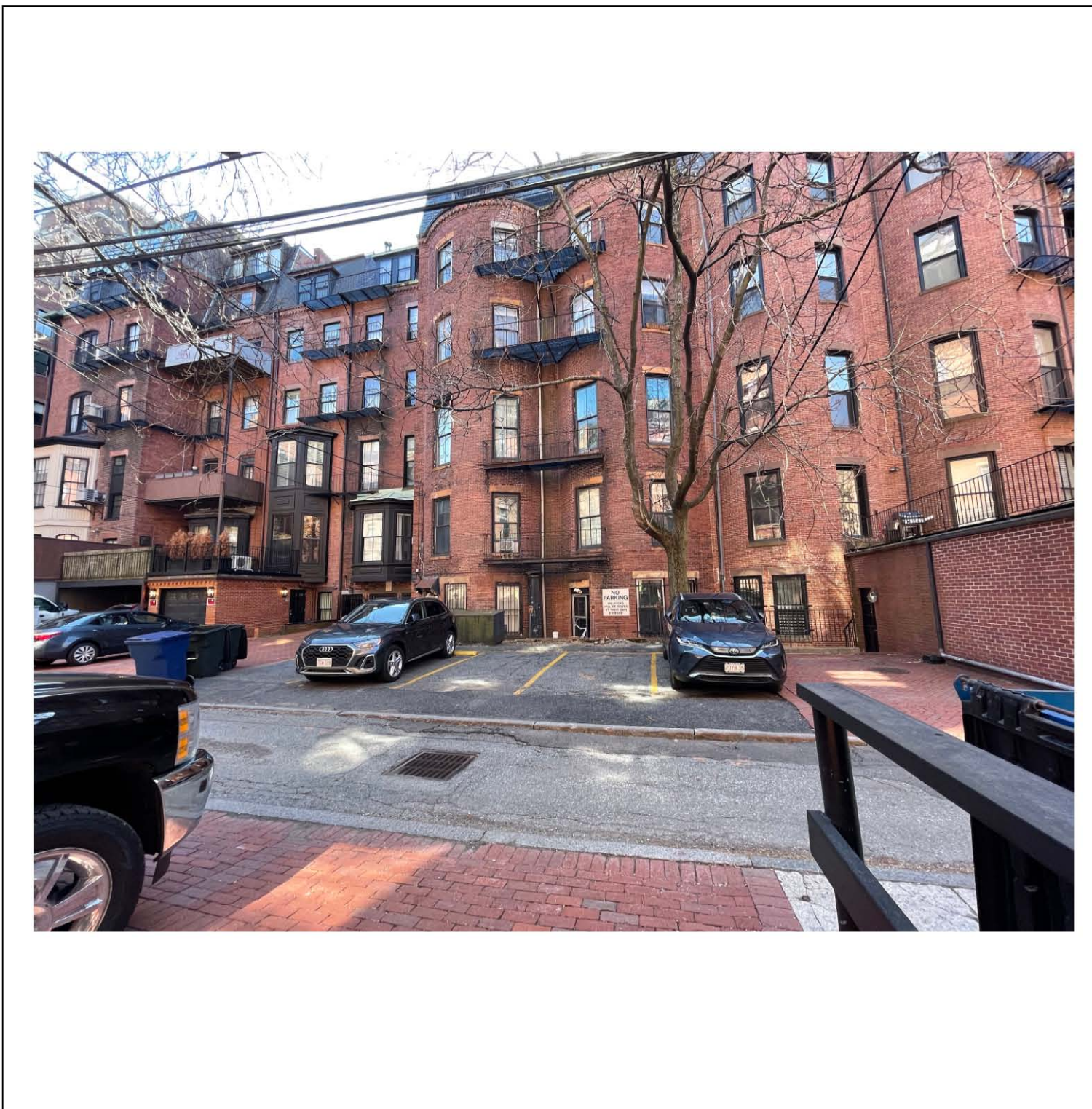
① PHOTO OF REAR ELEVATION
