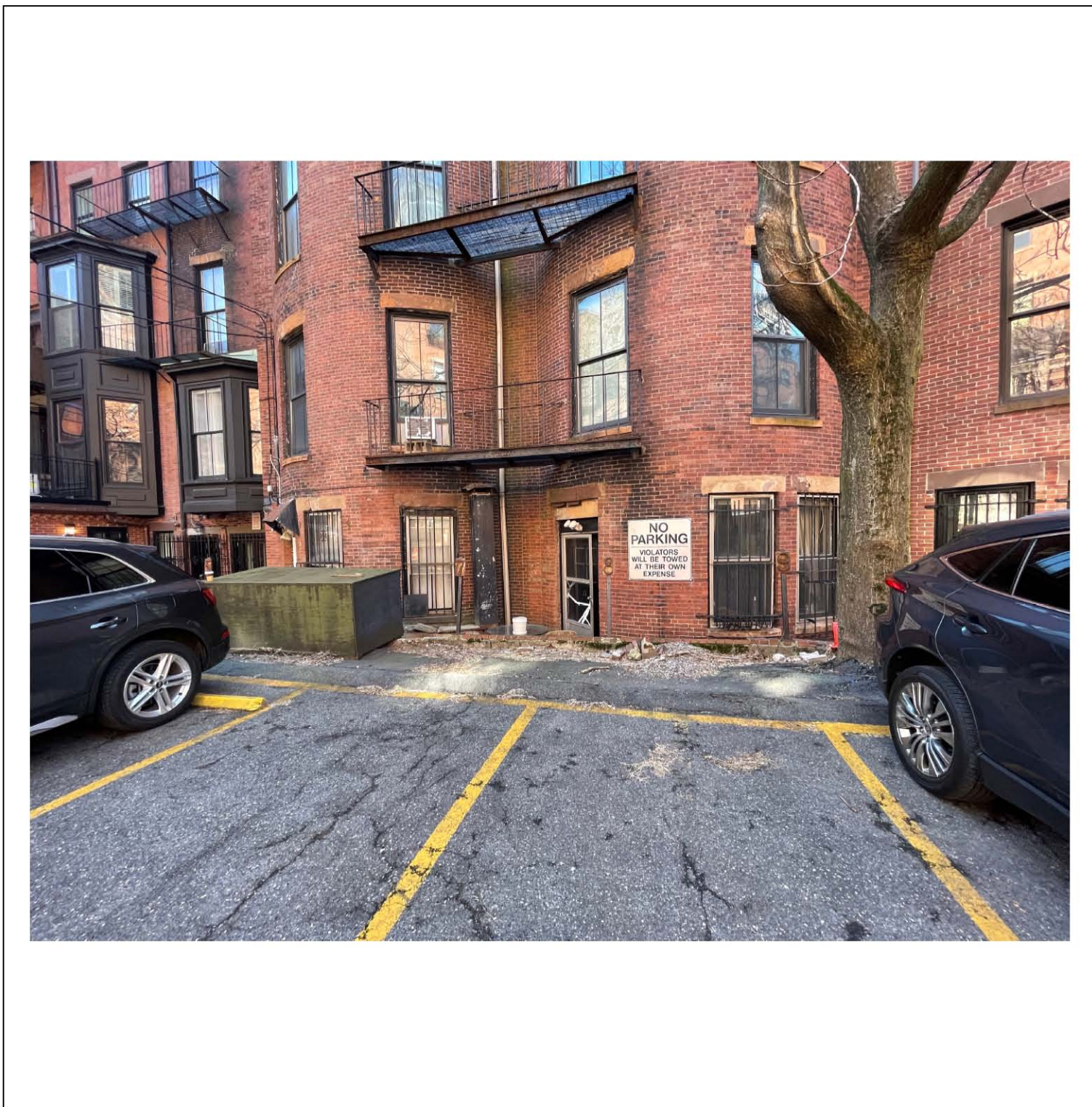
② PHOTO OF GROUND FLOOR REAR ELEVATION
