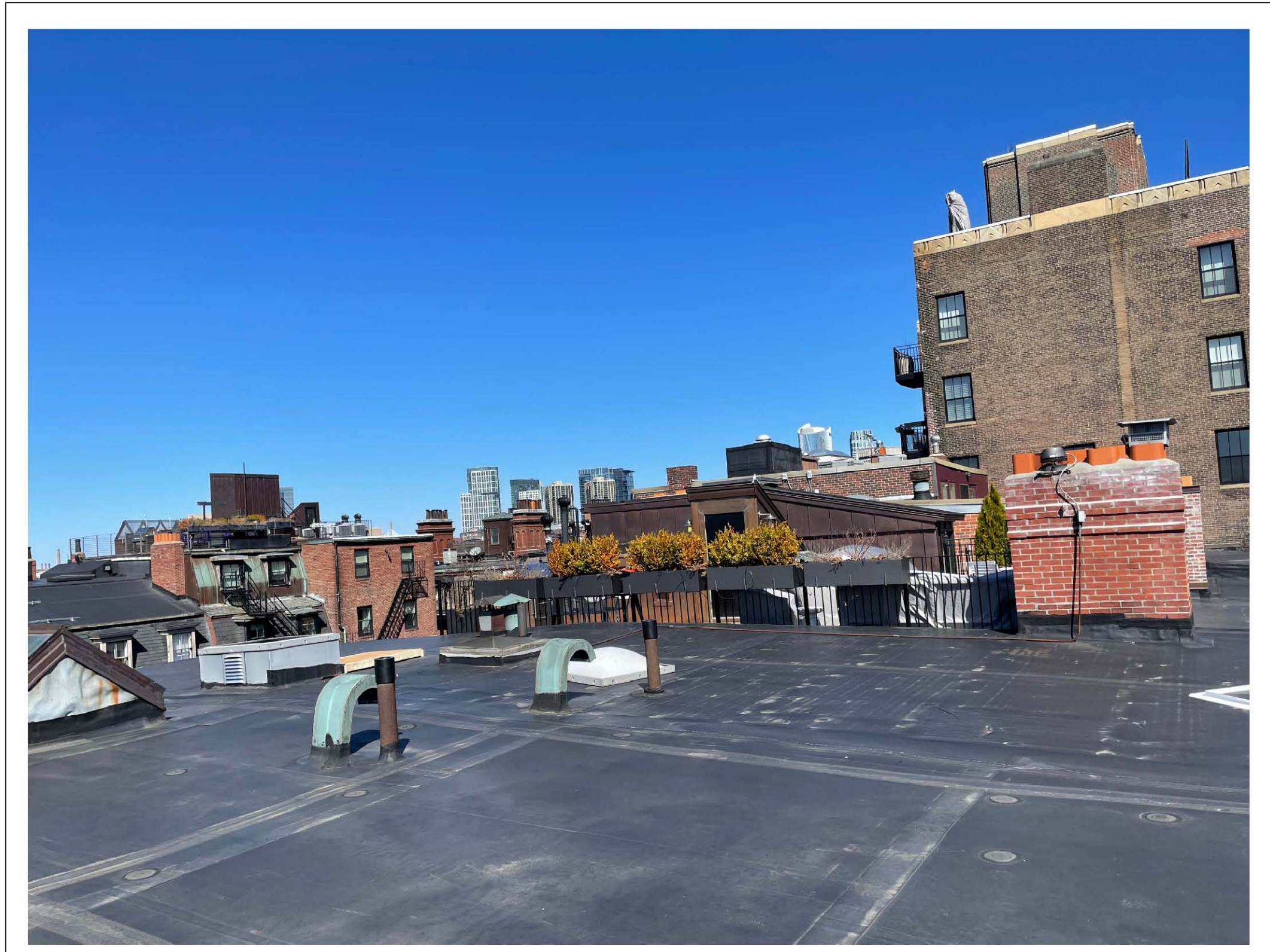
① PHOTO OF EXISTING ROOF LOOKING NORTH EAST
