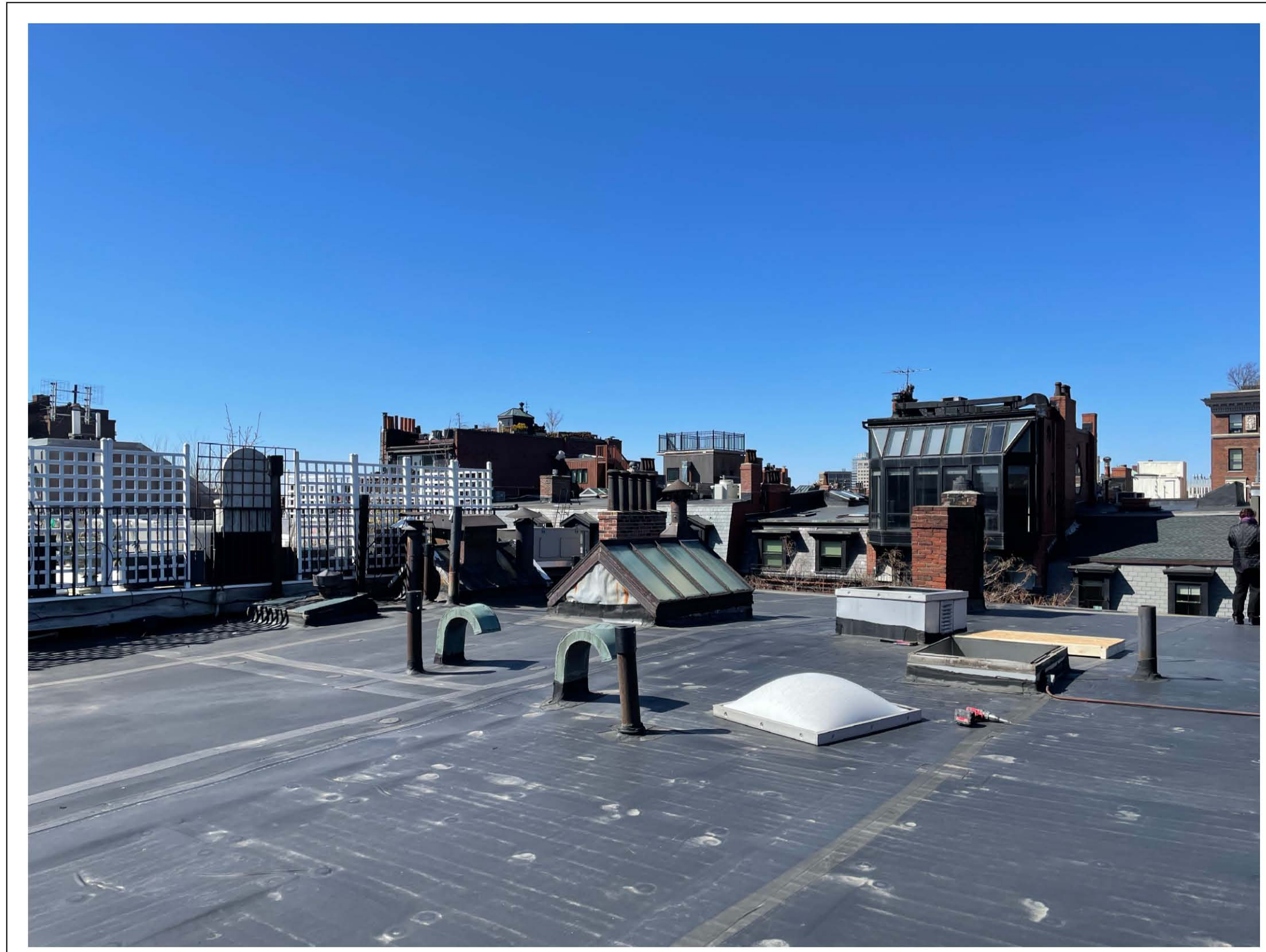
③ PHOTO OF EXISTING ROOF LOOKING NORTH WEST
