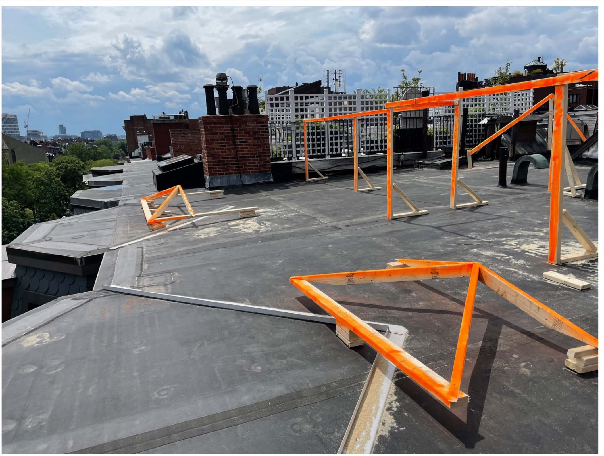
④ MOCK-UP OF SOUTH DECK RAIL AND SKYLIGHTS LOOKING WEST
