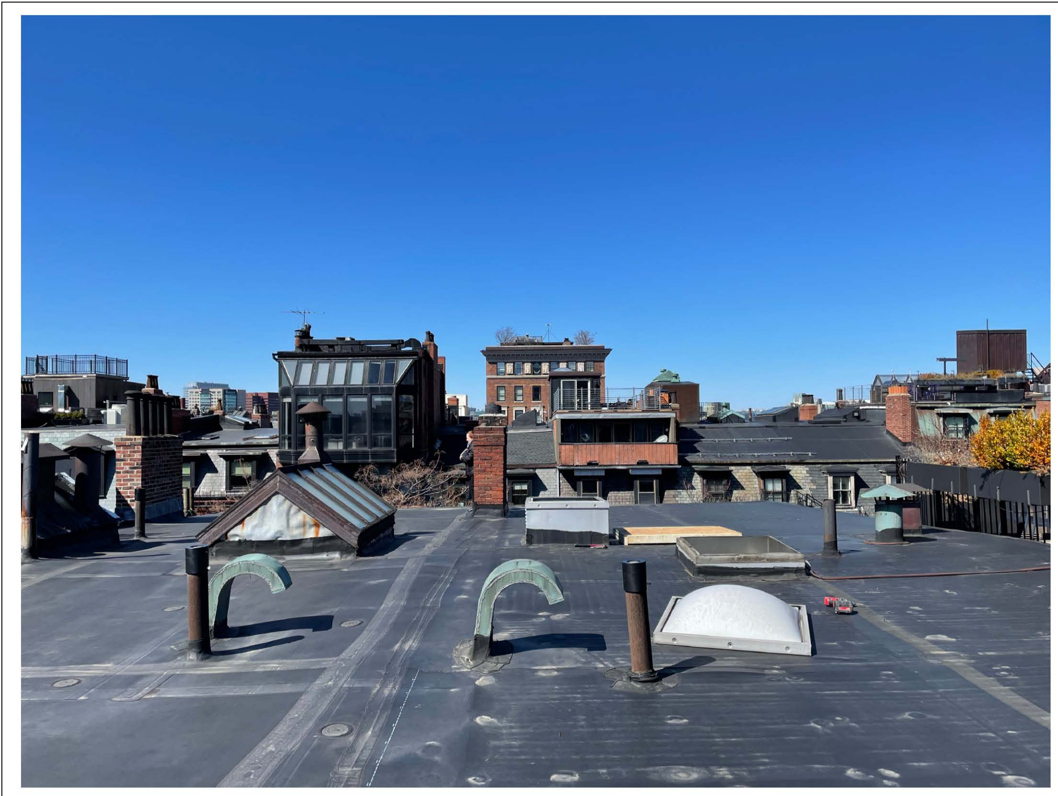
② PHOTO OF EXISTING ROOF LOOKING NORTH
