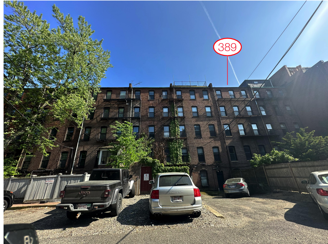
VIEW LOOKING SOUTH TOWARDS REAR OF BUILDING INCL. 381-383-385-387-389-391 MARLBOROUGH STREET (REAR FACADES)
