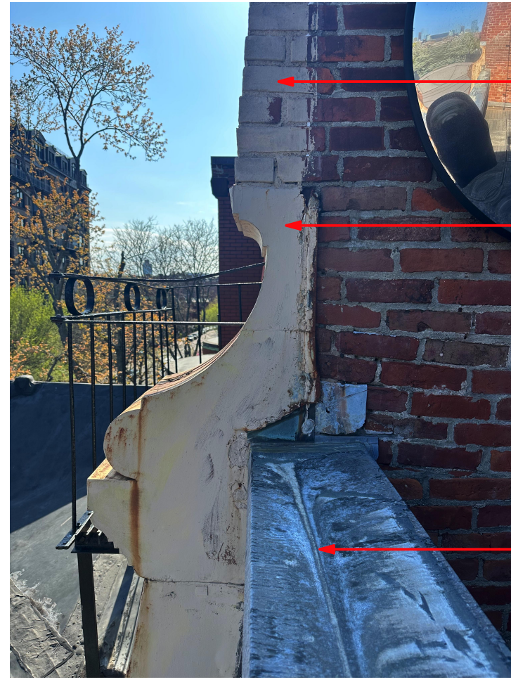
PENTHOUSE TERRACE - PARTY WALL DETAIL LOOKING WEST
