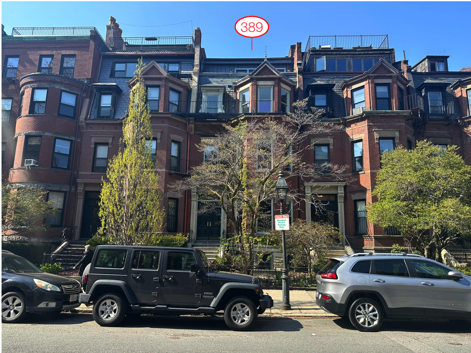
A Front Facade & Neighboring Context - Looking North From Marlborough Street
