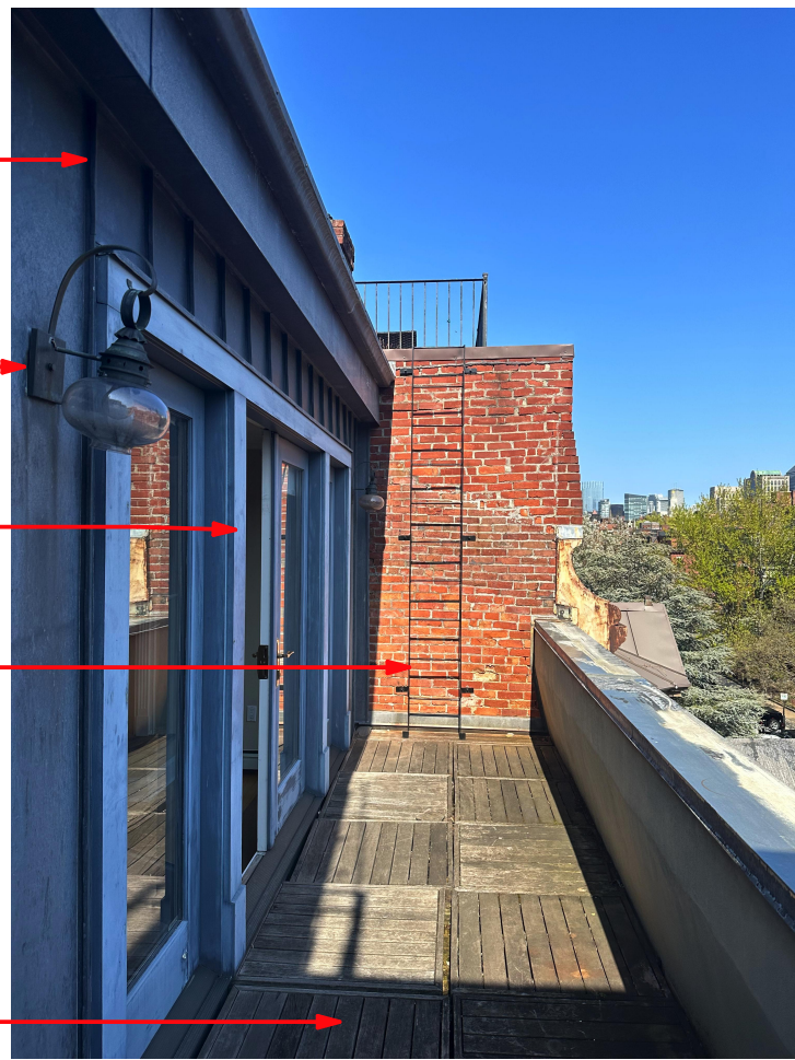
PENTHOUSE TERRACE LOOKING EAST
