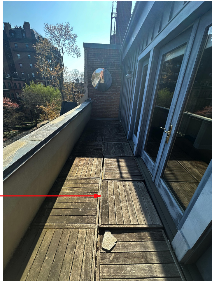
PENTHOUSE TERRACE LOOKING EAST
