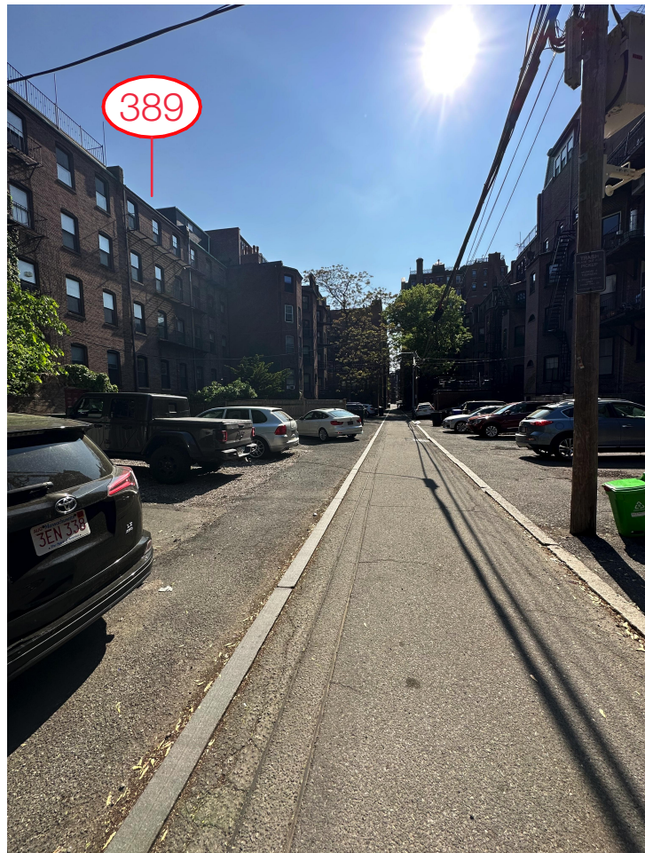
VIEW LOOKING WEST ALONG ALLEY
