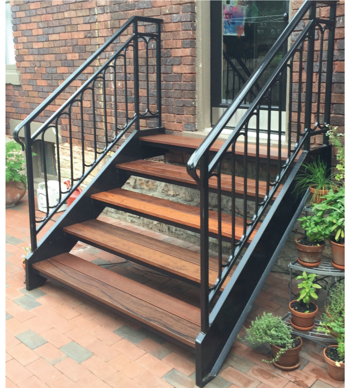
Steel Stringers and Wood Treads Open Riser Stairs
