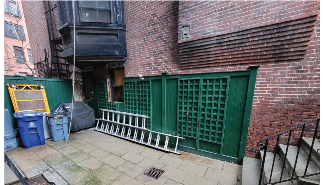
View 9 - Basement Glass Door to Neighbor
