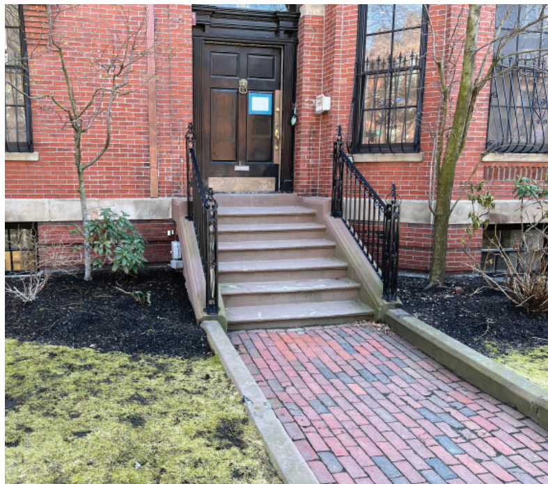
View 4 - Front Steps and Curb
