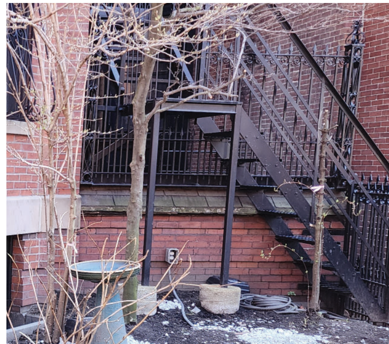
View 5 - Fire Escape Piers, Brick Wall
