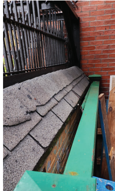
View 8 - Wood Cap Brick Wall
