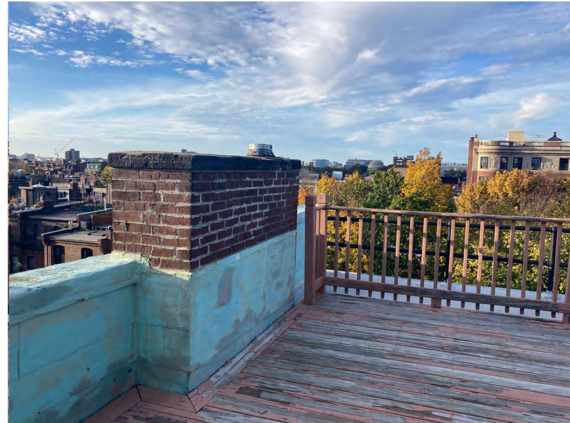
05 ROOF TOP - CURRENT CONDITION PHOTO 05 NOT TO SCALE
