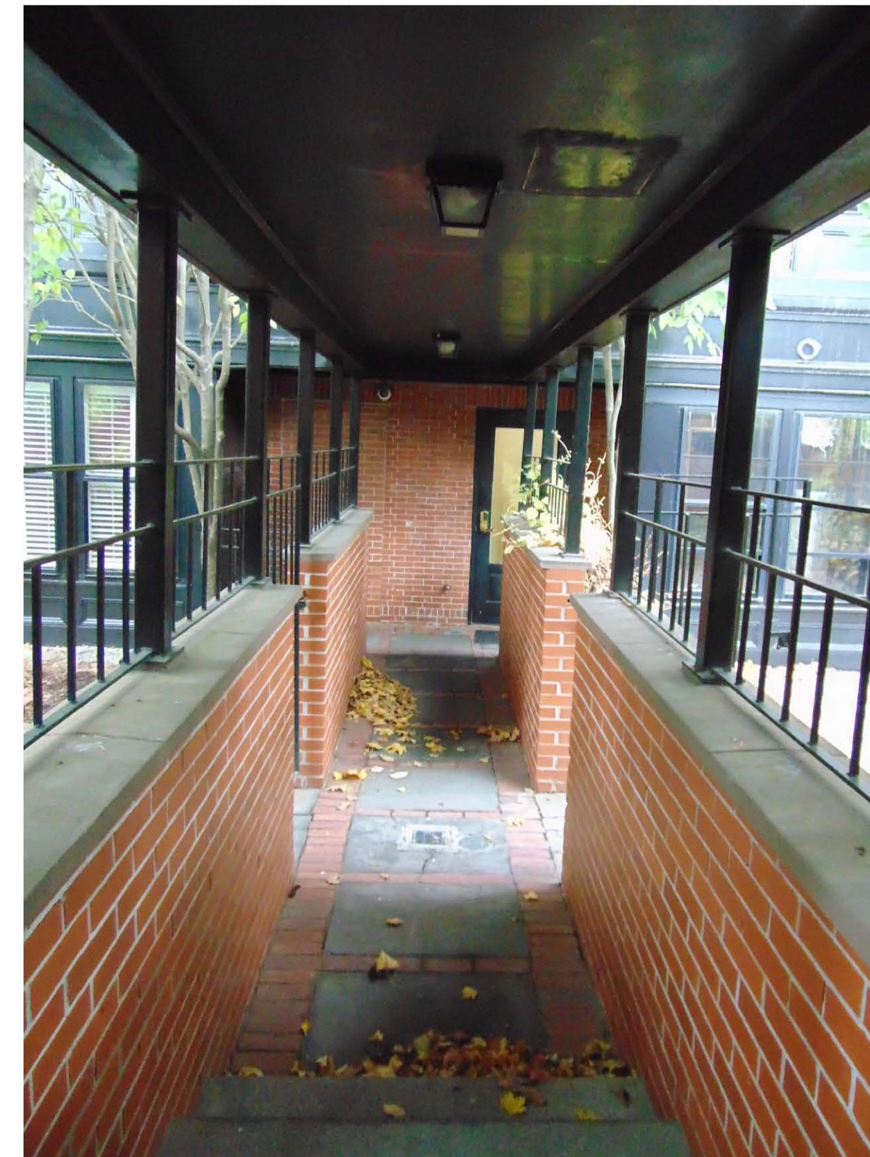
7 VIEW OF CONNCTOR LOOKING TOWARD BUILDING SCALE: No Scale
