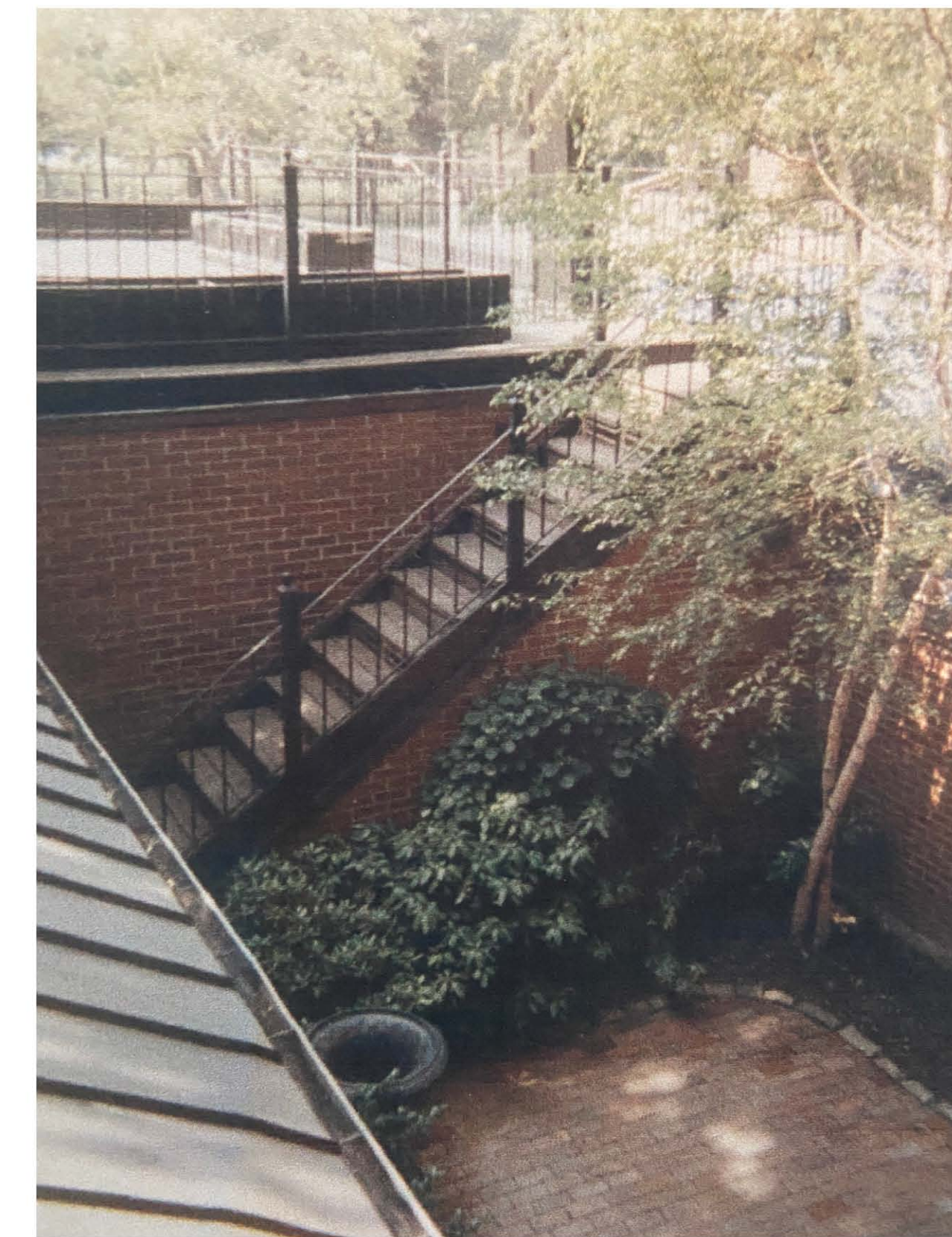
8 VIEW OF EXISTING STAIR TO DECK SCALE: No Scale
