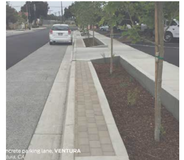
PERMEABLE PAVER STRIP
