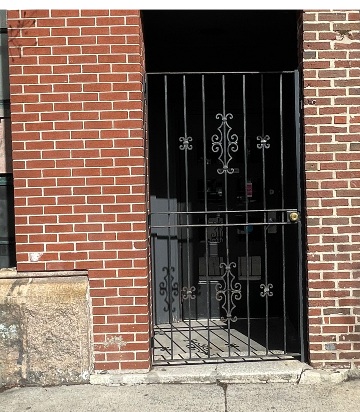
NOMINAL BRICK, FULL DEPTH, WITH MORTAR TO MATCH STANDARD SOUTH END BRICK PROFILES AND COLORS.
