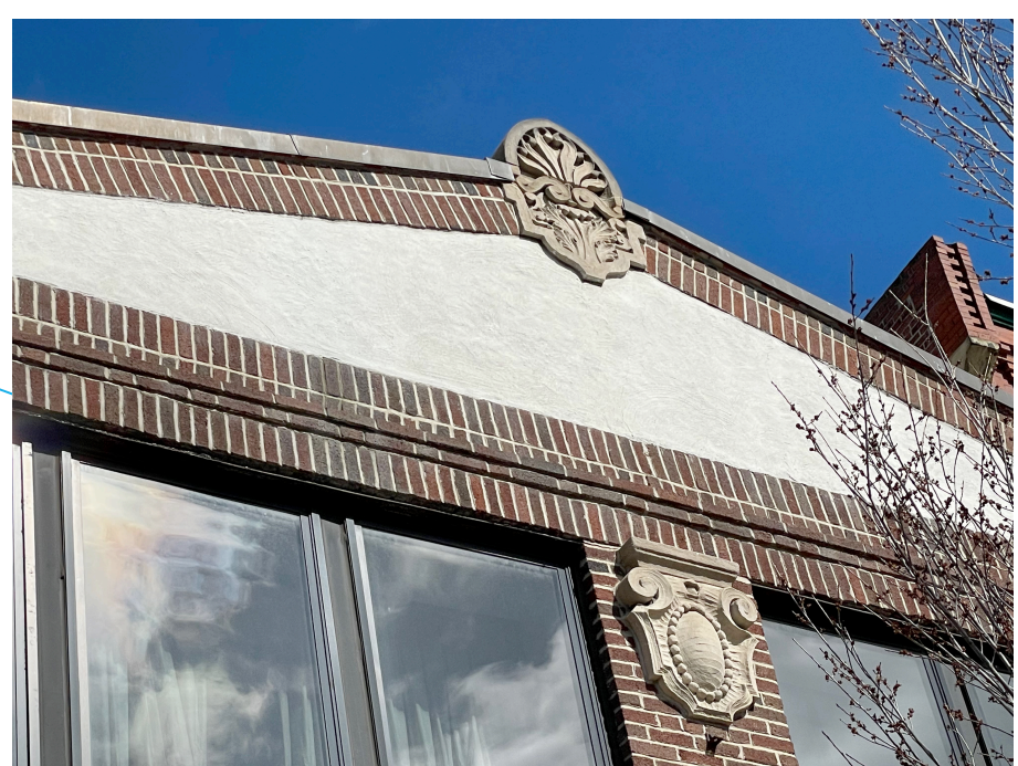
EXISTING PEDIMENT; STUCCO INFILL TO REMAIN
