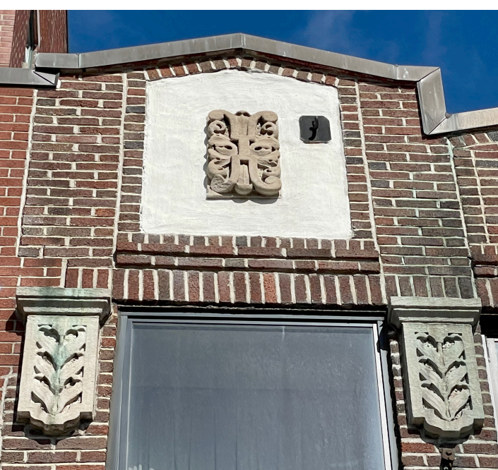
EXISTING CONCRETE ACCENT INLAY MEDALLIONS, CELANED AND REFERBISHED AS REQUIRED.
