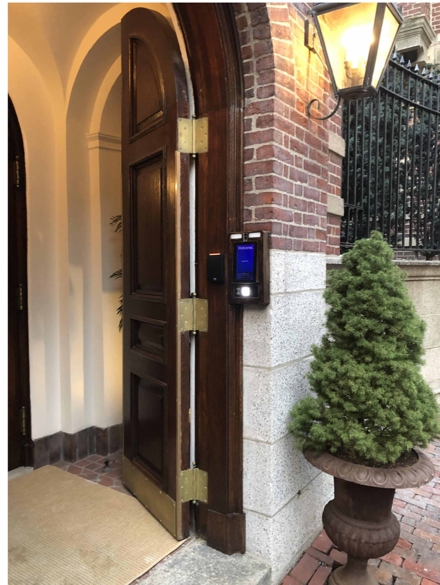
VIEW OF INTERCOM
