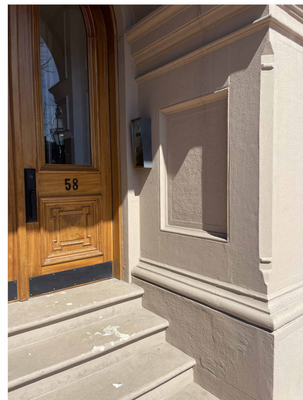
6 58 BEACON STREET EXISTING
