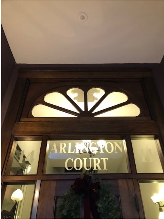
MAIN EXISTING DOOR - DOOR FRAME TO BE PAINTED
