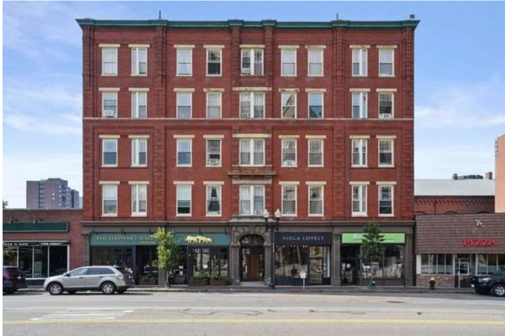
WASHINGTON STREET FACADE SHOWING MAIN RESIDENTIAL ENTRANCE
