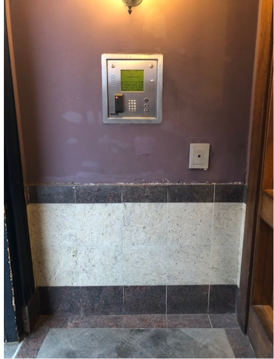
EXISTING CIRCA 1995 TILE TO BE REMOVED (WEST WALL)
