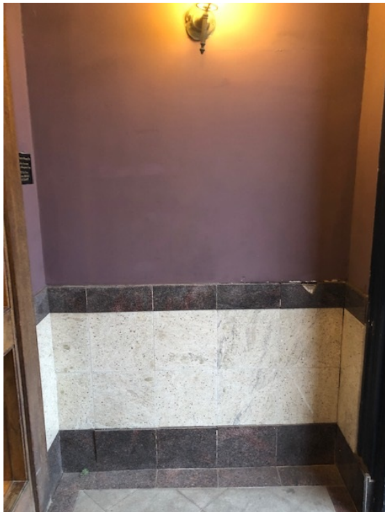
MAIN ENTRY DETAIL EAST WALL - TILE TO BE REMOVED
