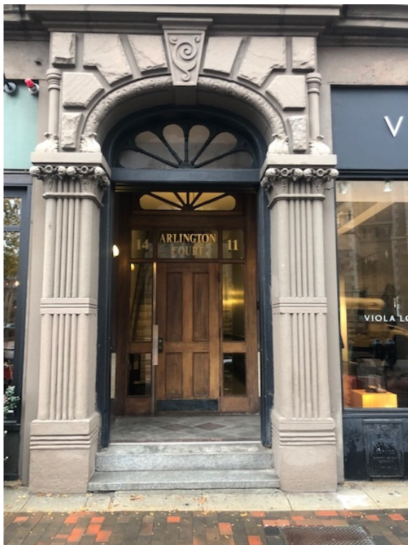
ENTRY PORTAL (HISTORIC)
