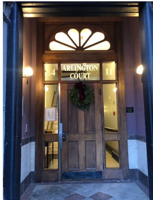
MAIN EXISTING DOOR W/ WAINSCOT TILE (NON-HISTORIC)
