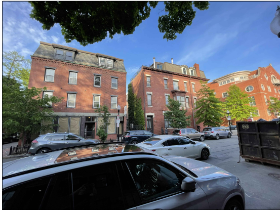
VIEW FROM CLARENDON LOOKING SOUTHEAST
