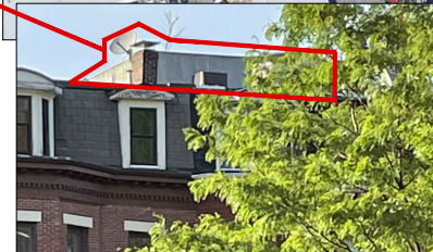
2 CLOSE UP OF VISIBLE ROOF DECK RAILING
