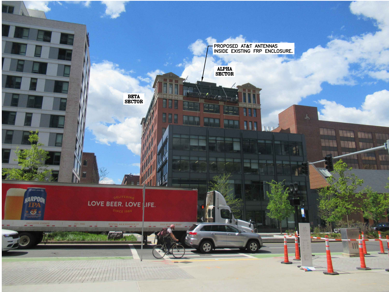
VIEW SOUTHWEST FROM SEAPORT BLVD
