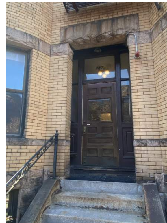
EXISTING PRECEDENT - 187 ST BOTOLPH
