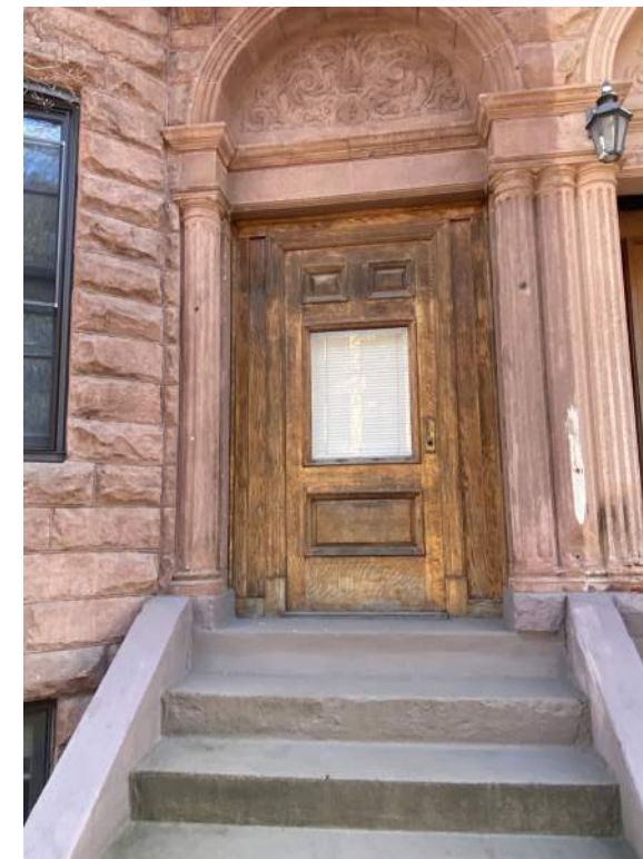
EXISTING PRECEDENT - 168 ST BOTOLPH
