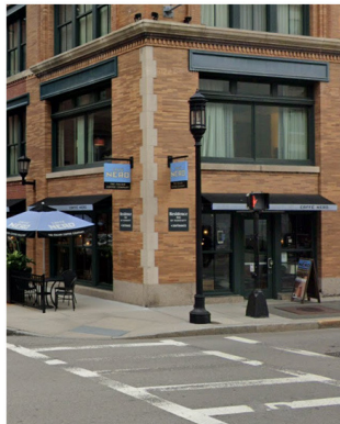
single light fixture
