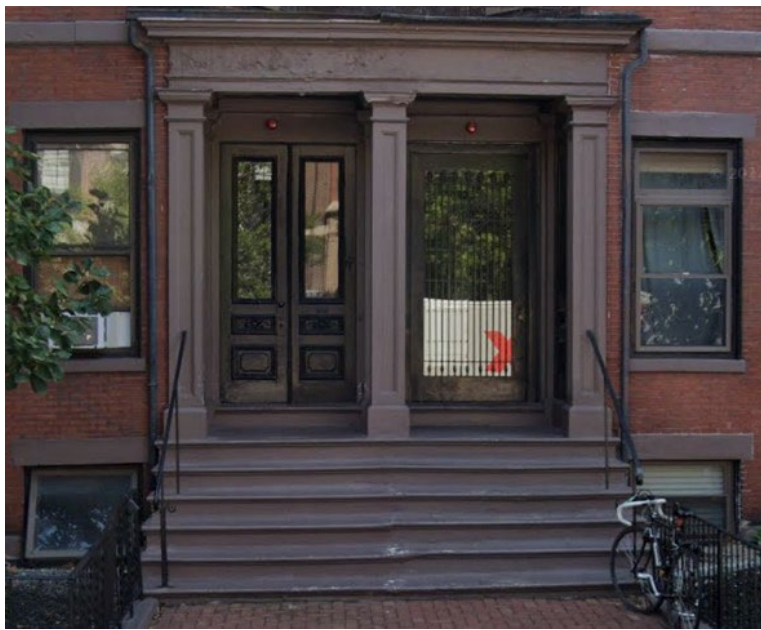
EXISTING FRONT ENTRY
