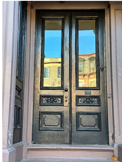
EXISTING DOOR AT 393 BEACON TO BE REPLICATED FOR 395 BEACON
