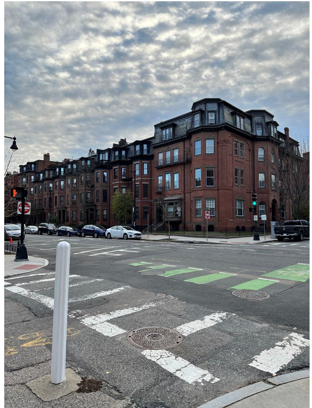
VIEW FROM GLOUCESTER STREET
