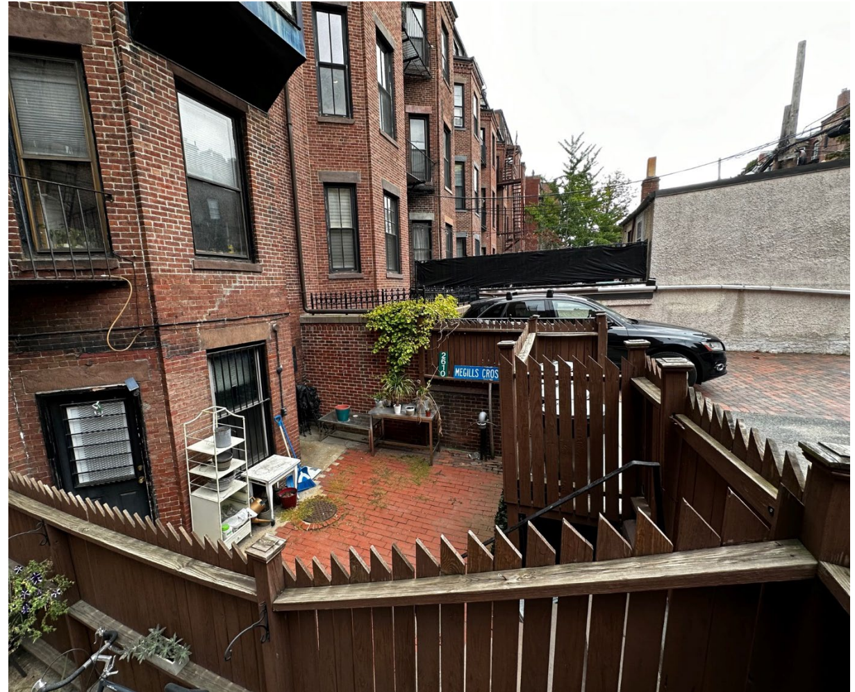
EXISTING SUNKEN GARDENS
