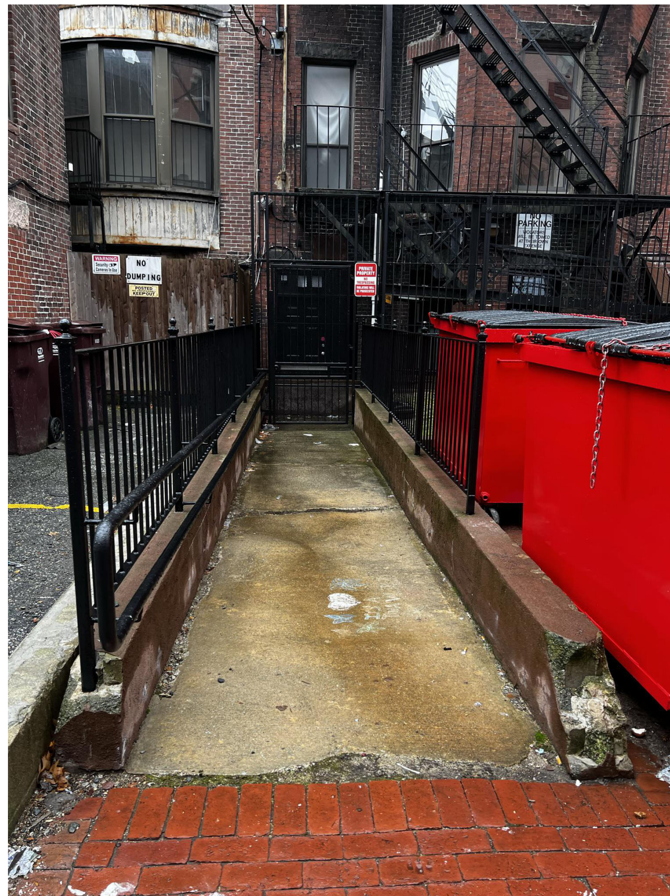
EXISTING RAMP TO BE REPLACED W/ CONCRETE PAVERS; WALLS TO BE REPAIRED; PARGED, AND PAINTED, SECOND HANDRAIL ADDED
