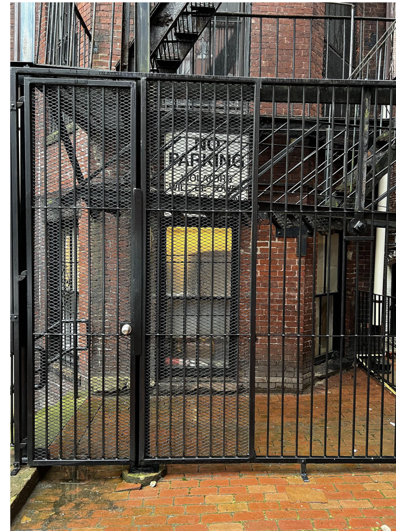
SECURITY GATE AND 'NO PARKING' SIGNS TO BE REMOVED
