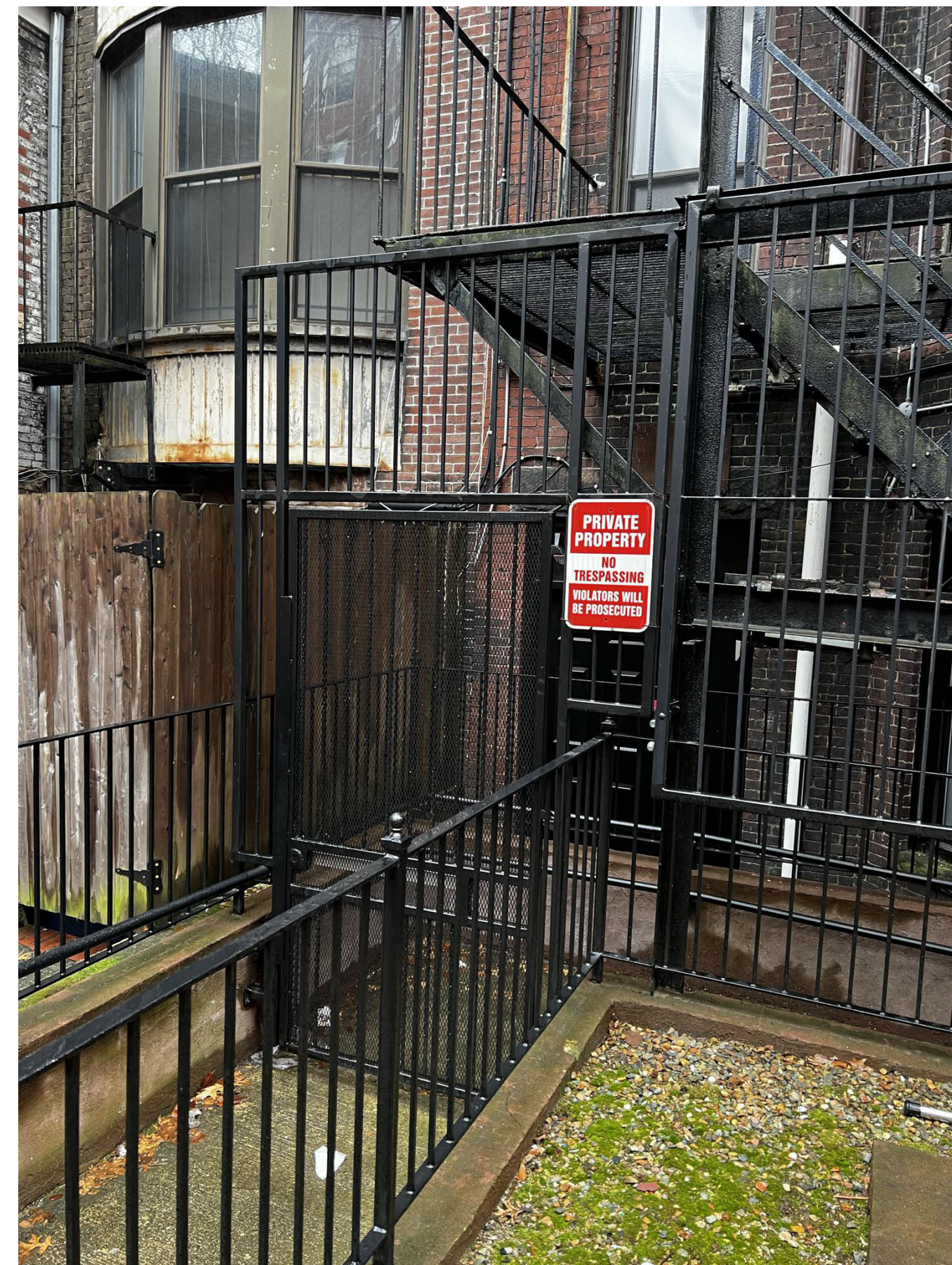
SECURITY GATE TO BE REMOVED
