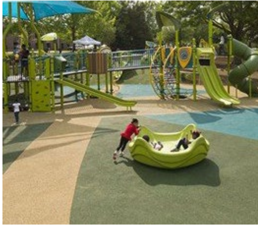
Poured-in-place (PIP) Rubber Surfacing
