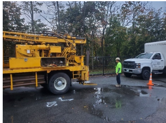
Photo 2: View of truck drill rig at boring location NB-1.
