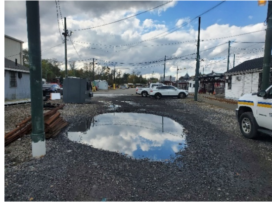
Photo 1: View of MBTA Mattapan Station Parking lot, from boring location NB-3.
