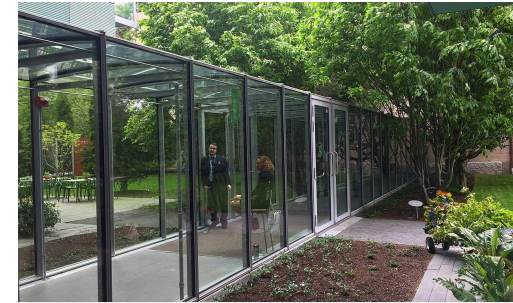
Indoor connection to pool
