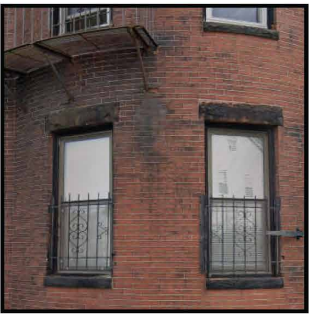
HALF-BARS & LOW YARD RAILINGS
