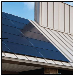
STANDING SEAM SLOPED ROOF
