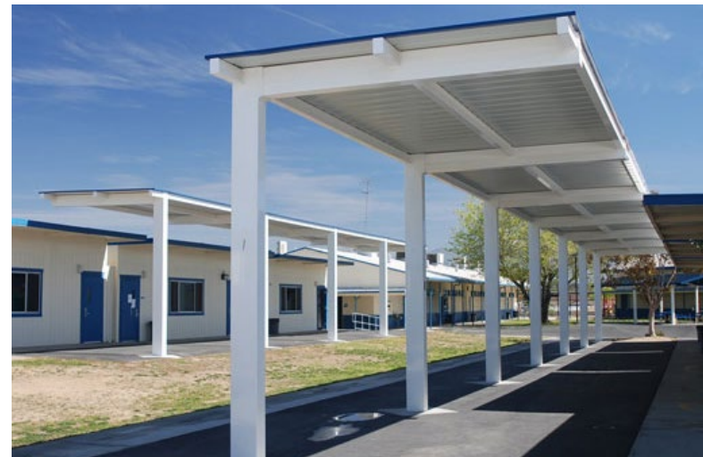
Cantilever – fully covered
