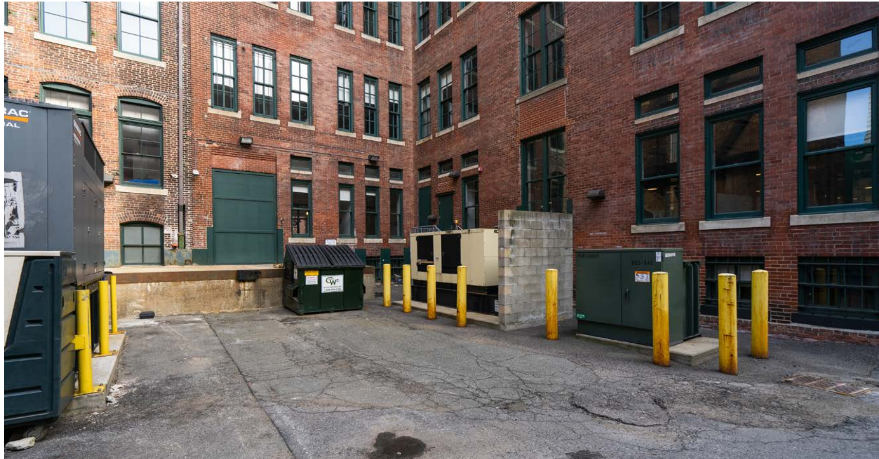
EXISTING VIEW OF 51 MELCHER FROM NECCO COURT
