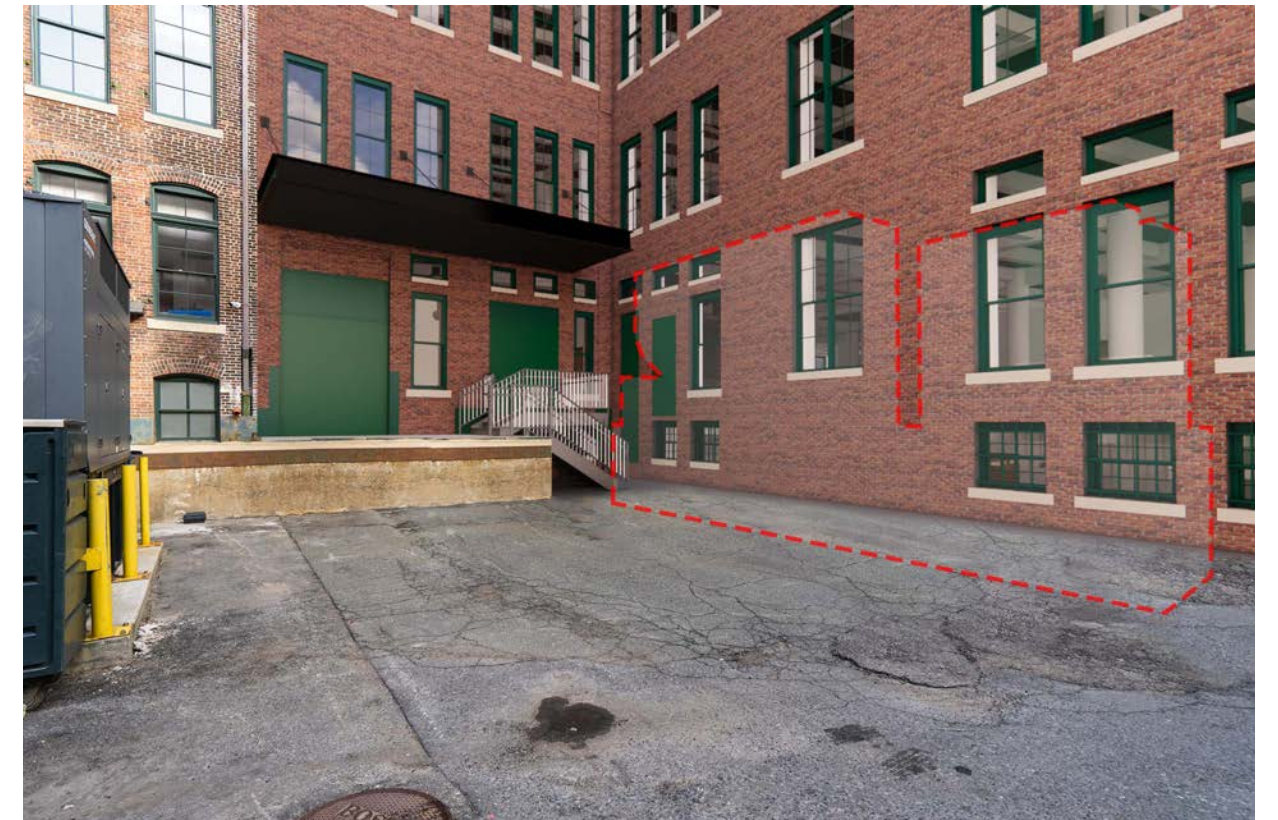
PREVIOUSLY APPROVED VIEW WITH HIDDEN GENERATOR
