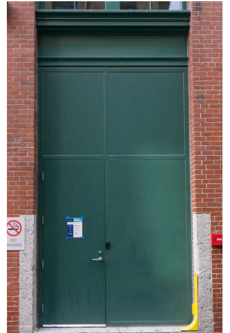
EXAMPLE OF METAL PANEL INFILL AND DOORS
