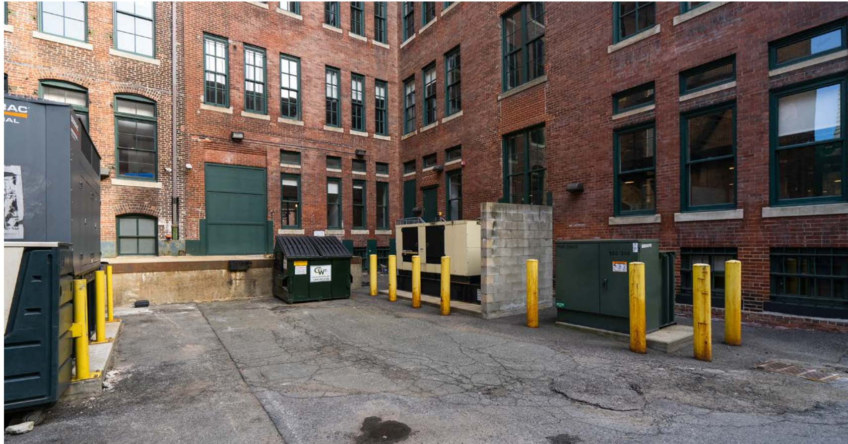
EXISTING VIEW OF 51 MELCHER FROM NECCO COURT
