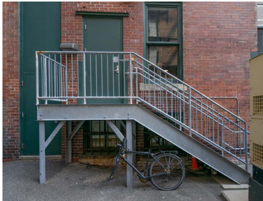
EXISTING STAIR TO BE REMOVED
