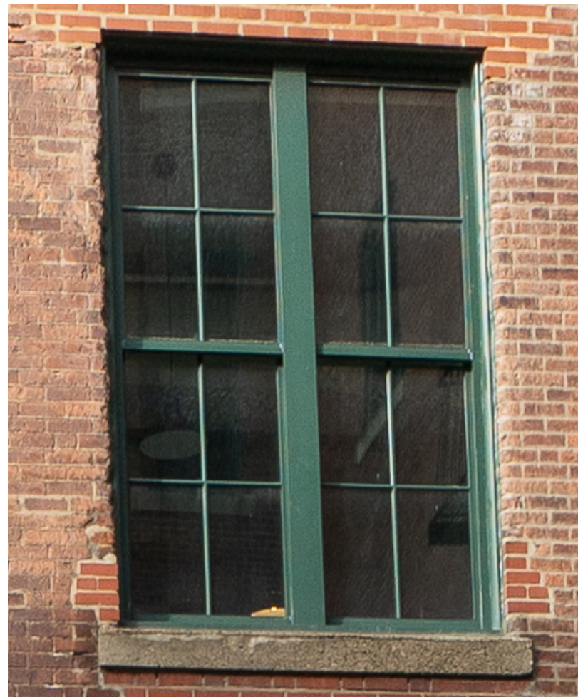
EXISTING WINDOW TO BE INFILLED
