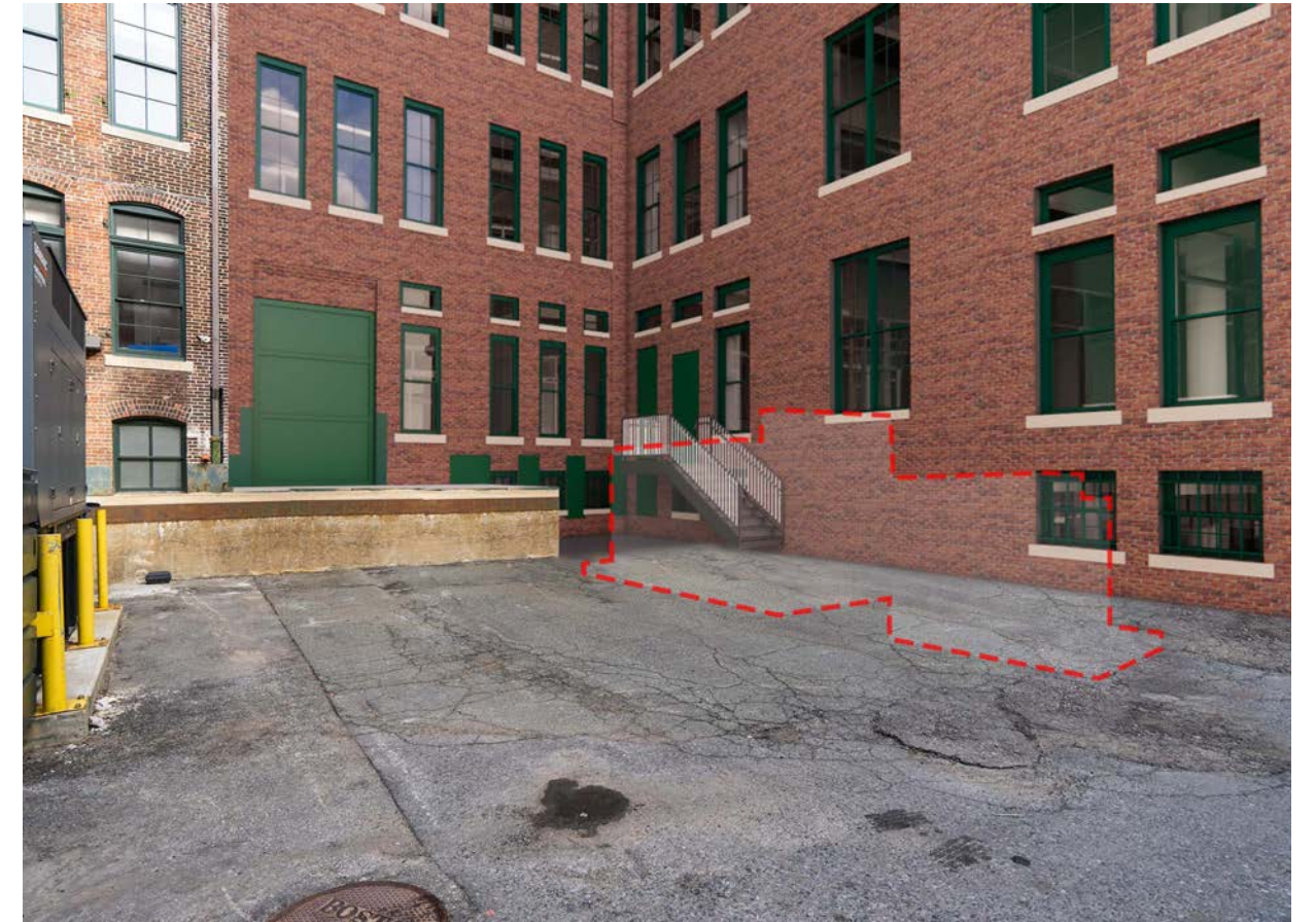
EXISTING VIEW WITH HIDDEN GENERATOR
