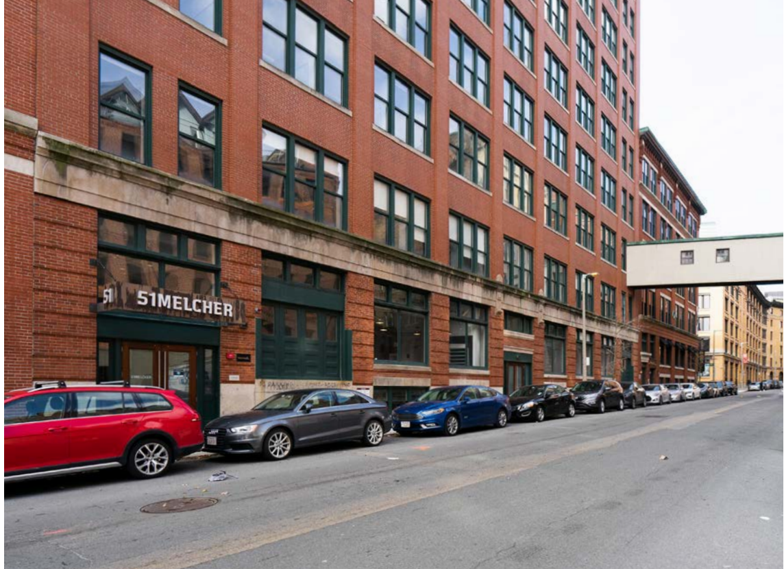
FRONT VIEW ON MELCHER ST
