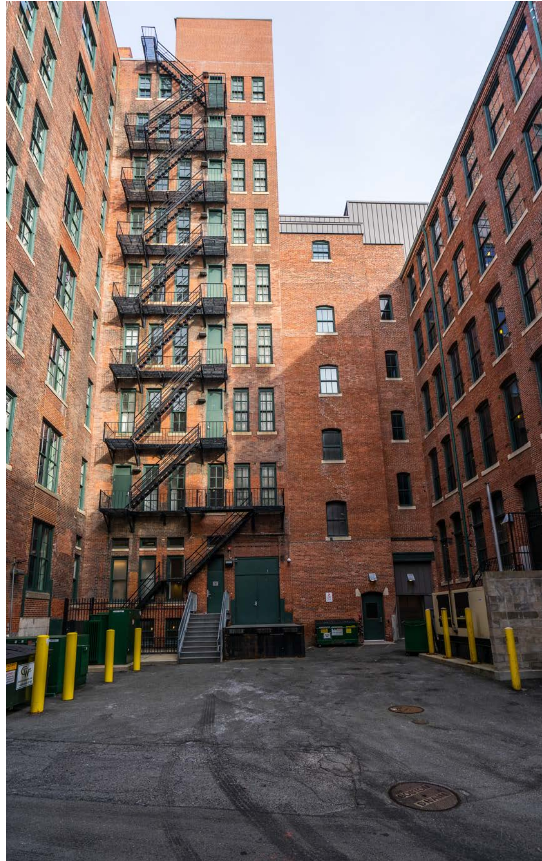
EXISTING LOADING DOCK
