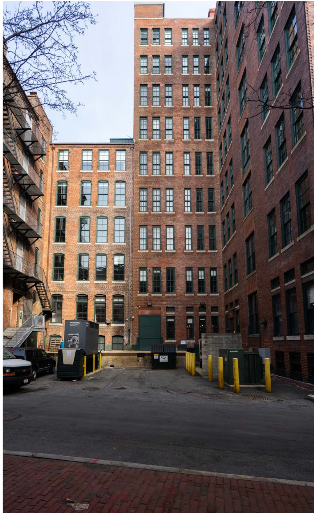
REVITALIZED LOADING DOCK
