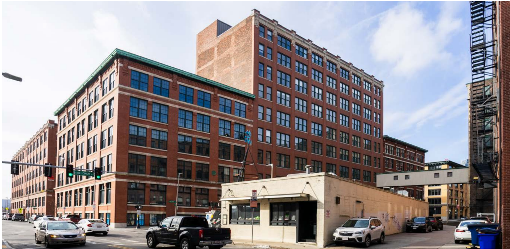
EXISTING VIEW OF 51 MELCHER FROM A ST
