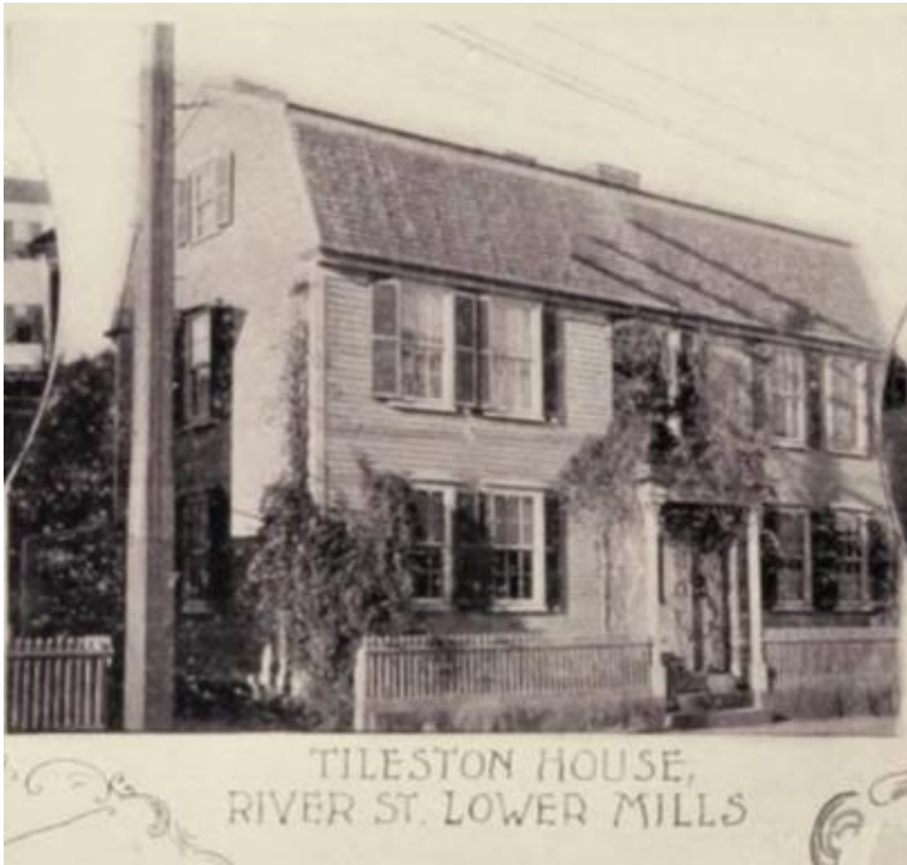
Figure 7. A late nineteenth-century photograph of 13 River Street, showing columns supporting entry porch roof, six-over-six windows with projecting surrounds, and chimney placement (Branch Alliance of Christ Church Unitarian (Christ Church). The Dorchester Book . Boston, MA: George H. Ellis, Printer, 1899).
