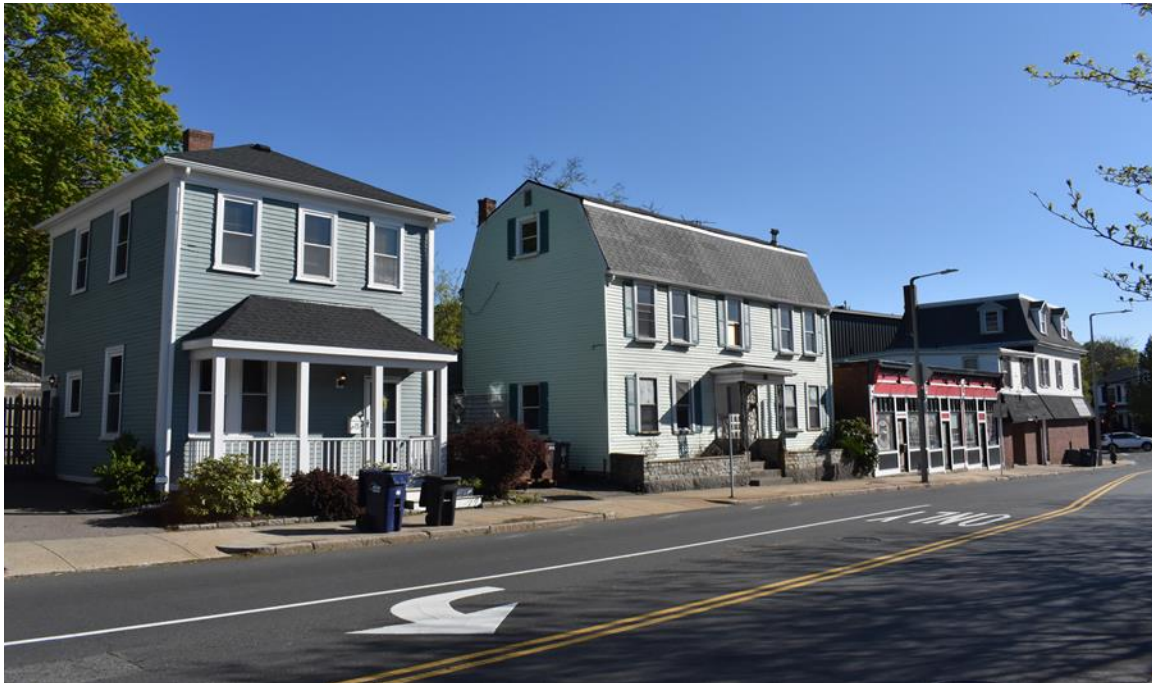
Figure 5. Front (south) and west elevations, view northeast along River Street toward Washington Street. Charles Tileston's tin shop was in the far right, Second Empire-style building, 1141 Washington Street (The Public Archaeology Laboratory, Inc. 2021).
