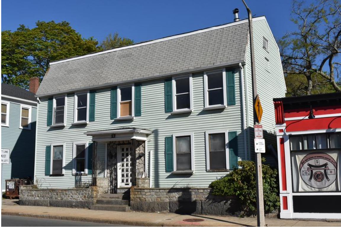
Figure 4. Front (south) and east elevations (The Public Archaeology Laboratory, Inc. 2021).
