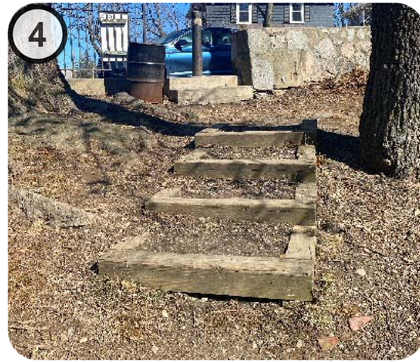
4 CONCRETE STAIRS AND WOOD STEPS IN FAIR CONDITION @ RICHVIEW ST. N.
