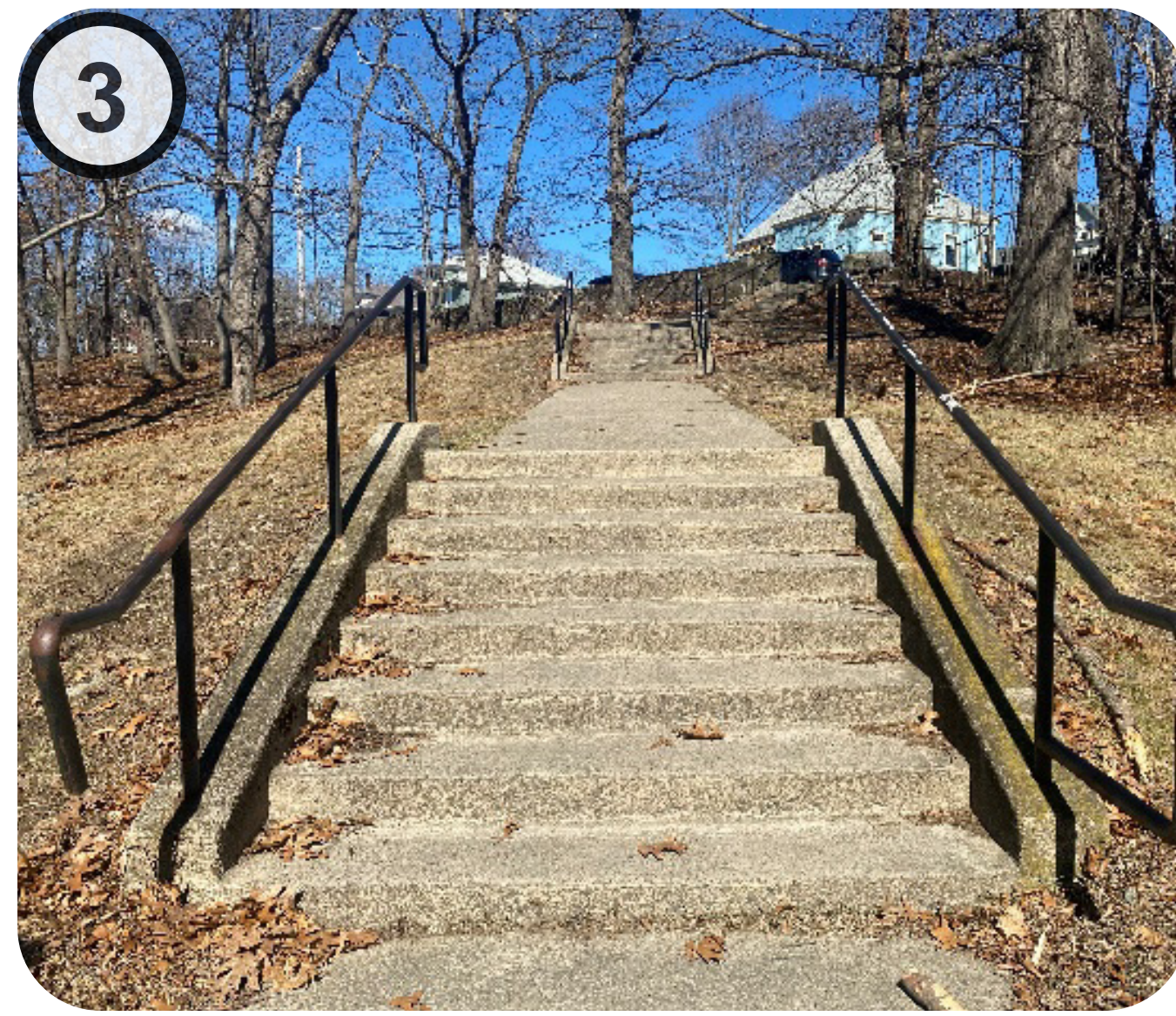
3 CONCRETE STAIRS WITH HANDRAILS IN FAIR CONDITION @ RICHVIEW ST. S.
