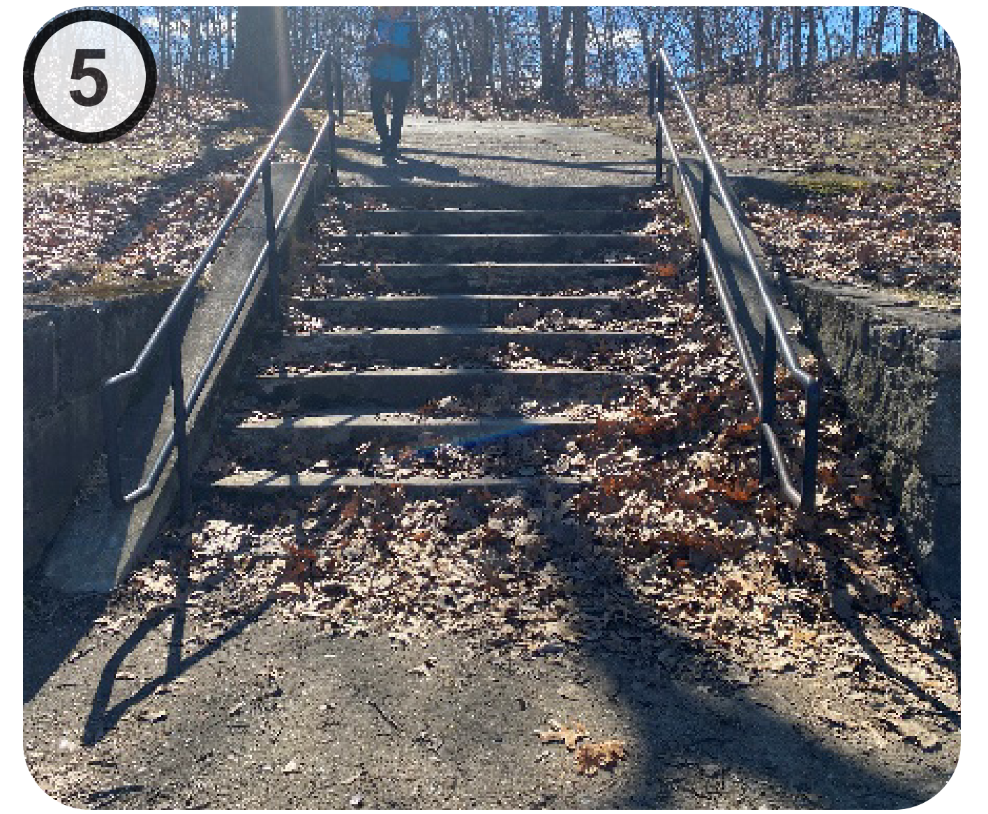
5 CONCRETE STAIRS W/ HANDRAILS IN FAIR CONDITION @ SOFTBALL COURT
