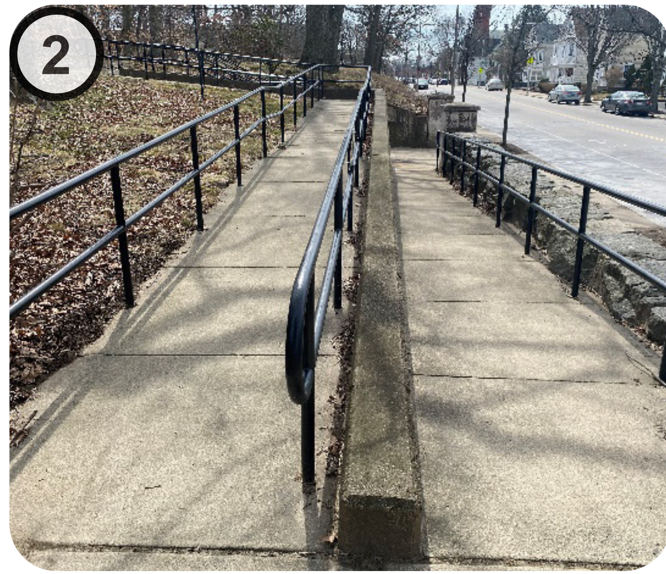
2 CONCRETE RAMPS WITH HANDRAILS IN FAIR CONDITION @ DORCHESTER AVE.
