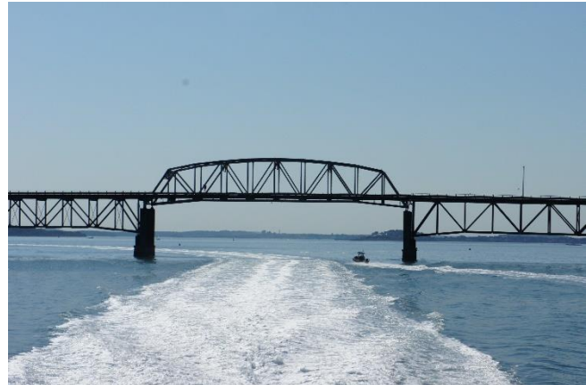
Navigation span of originally permitted bridge
