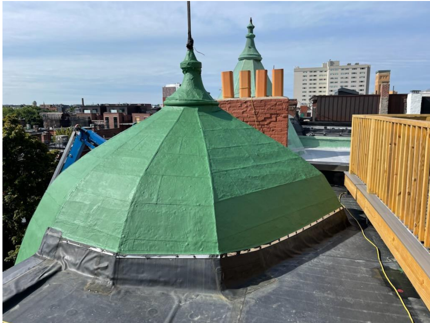
Photo 11: New coating application on dome roof.
