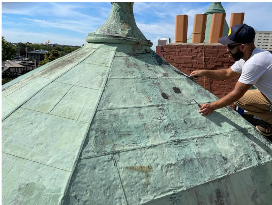
Photo 10: Contractor removing loose sections of coating and asphalt.
