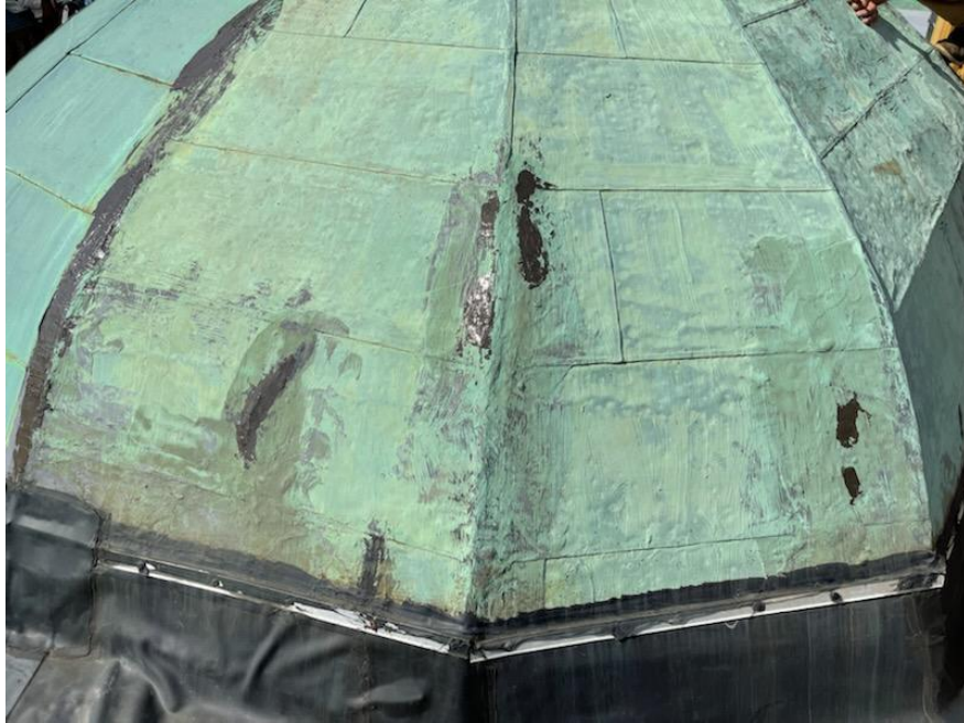
Photo 9: During prep work, loose sections of coating and asphalt required removal.
