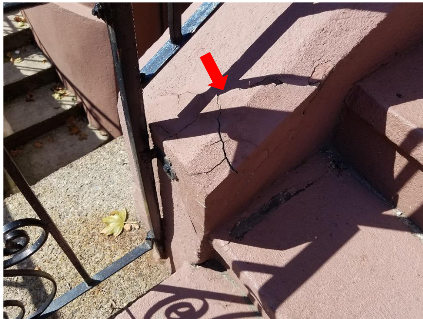
Photo 4: Perform random masonry repairs to defective concrete at front entrance stairway.
