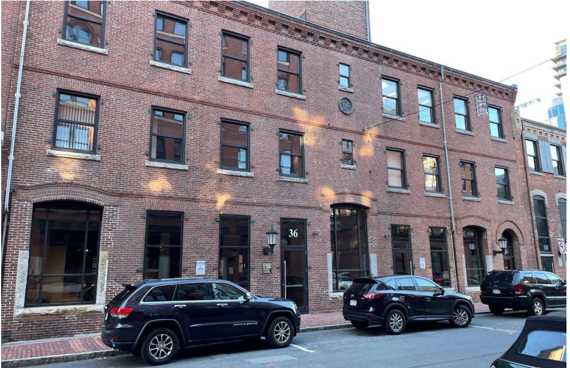
EXISTING CONDITION PHOTO
