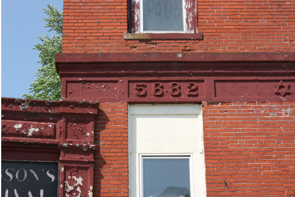
Figure 14. Façade detail of Roxbury Hebrew School. May 2022.
