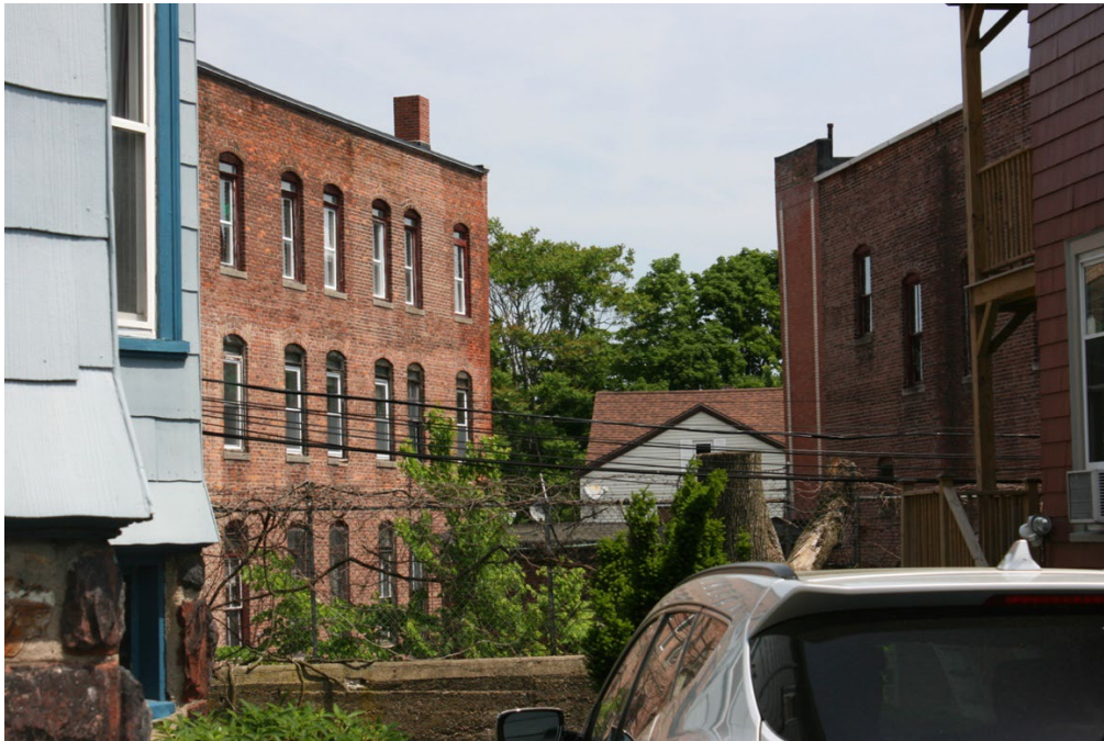
Figure 15. Courtyard elevations of Mt. Calvary Holy Church/Congregation Shara Tfilo Synagogue (R) and Roxbury Hebrew School (L). May 2022.
