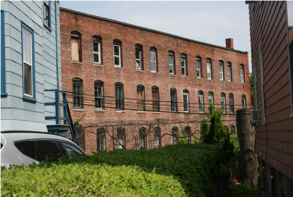
Figure 13. Southeast (courtyard) elevation of Roxbury Hebrew School. May 2022.
